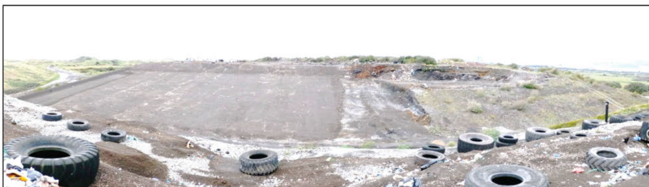
Figure 5 Photograph showing eastern flank of cell 1. Left hand side shows area of flank already re-profiled.
