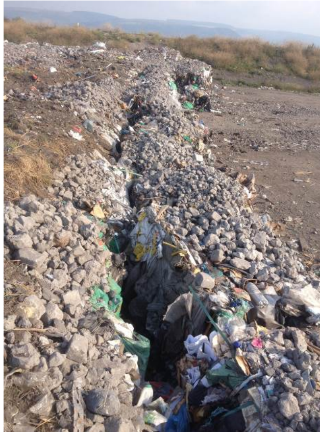
Plate 4-1 Gaps between bales in bio cell
