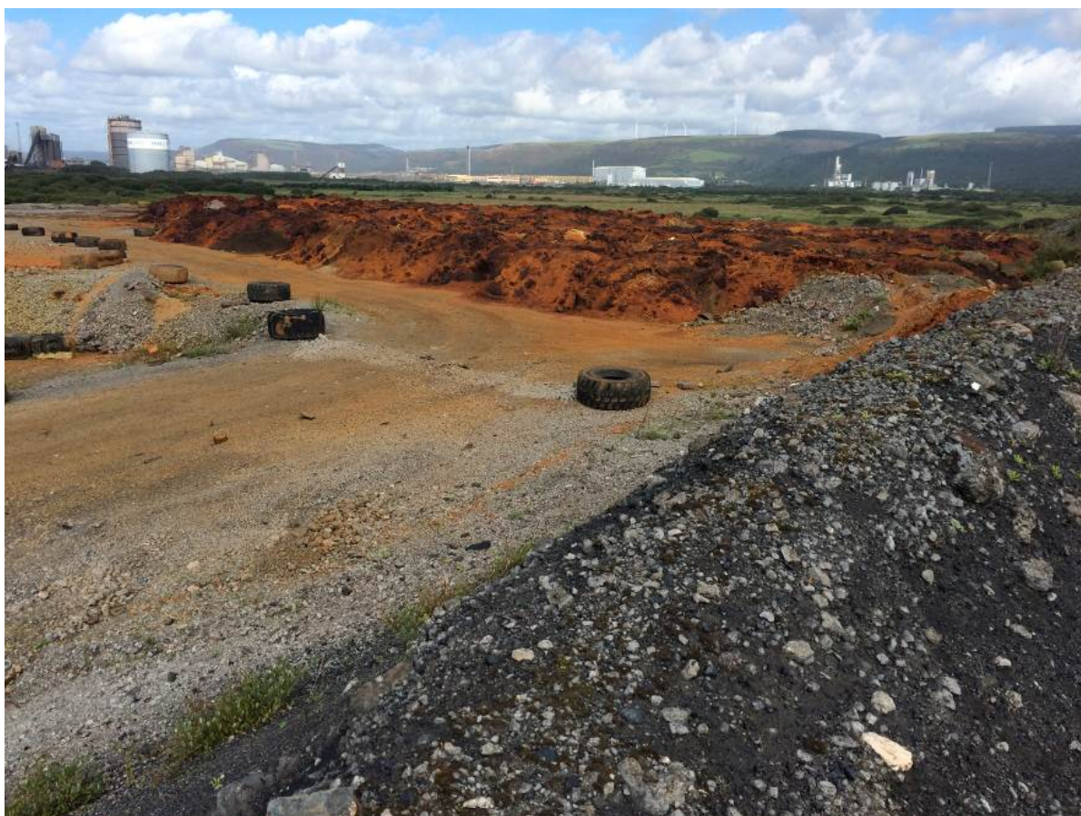
Plate 6-2 View North over MNHL Cell 2. Note dominance of iron rich filter cake
