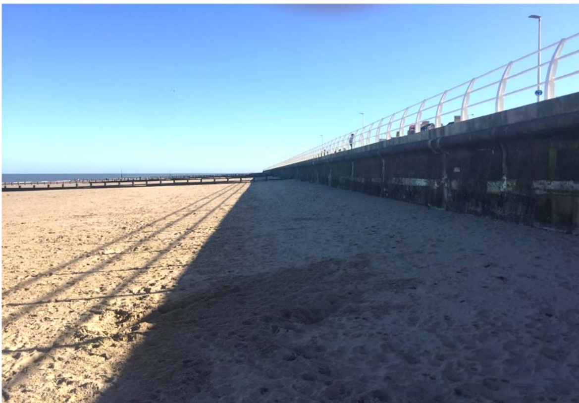
Figure 1-2: An example of current coastal protection at Central Rhyl
