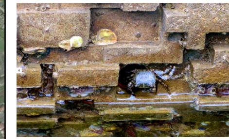
Opportunity to create habitats for rocky shore species by integrating prefabricated bio-blocks within rock armour defences, and textured concrete to stepped revetment
