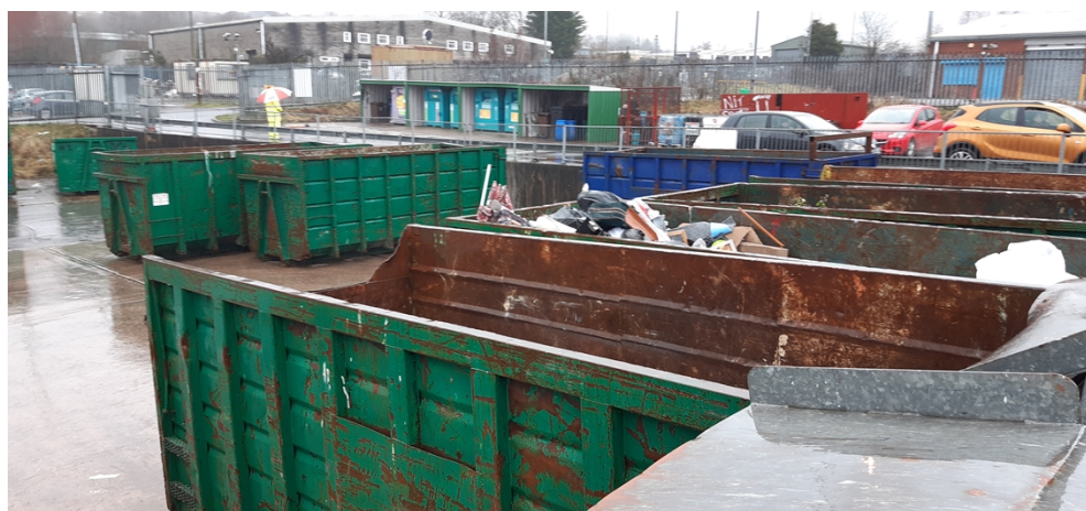
Photo 2 - Flooring condition along with segregated skips along with good housekeeping standards
