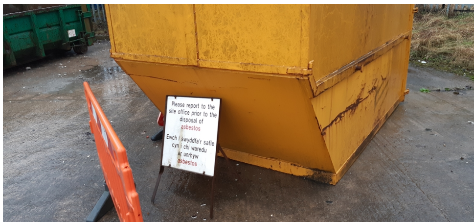
Photo 4 - Sealed skip containing asbestos waste
