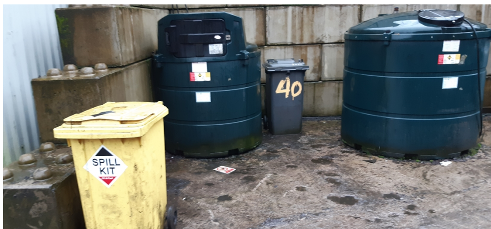
Photo 5 - Storage containers where waste fluids from cars are stored
