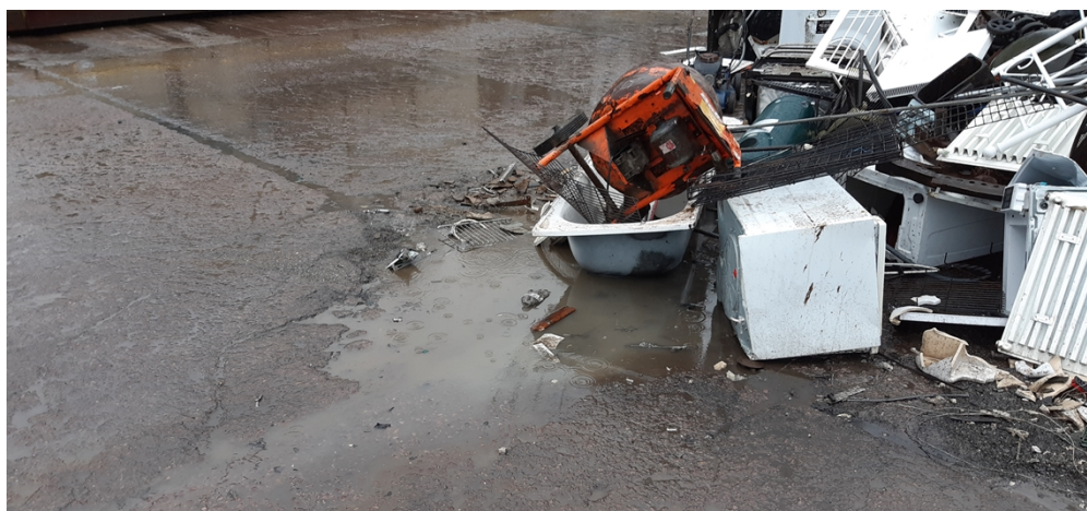
Photo 2 - Damaged flooring next to scrap metal waste stockpile
