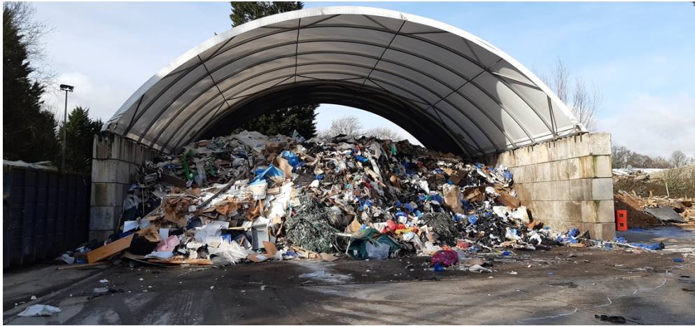
Photo 3 - General waste located underneath 'Zap' Shelter
