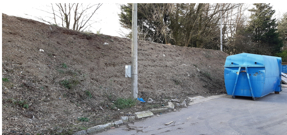
Photo 5 - Increased size of bund to assist with noise suppression on site
