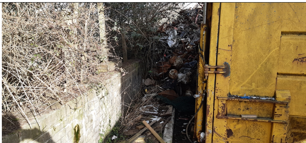
Photo 8 - No clear separation distance between waste and site boundary
