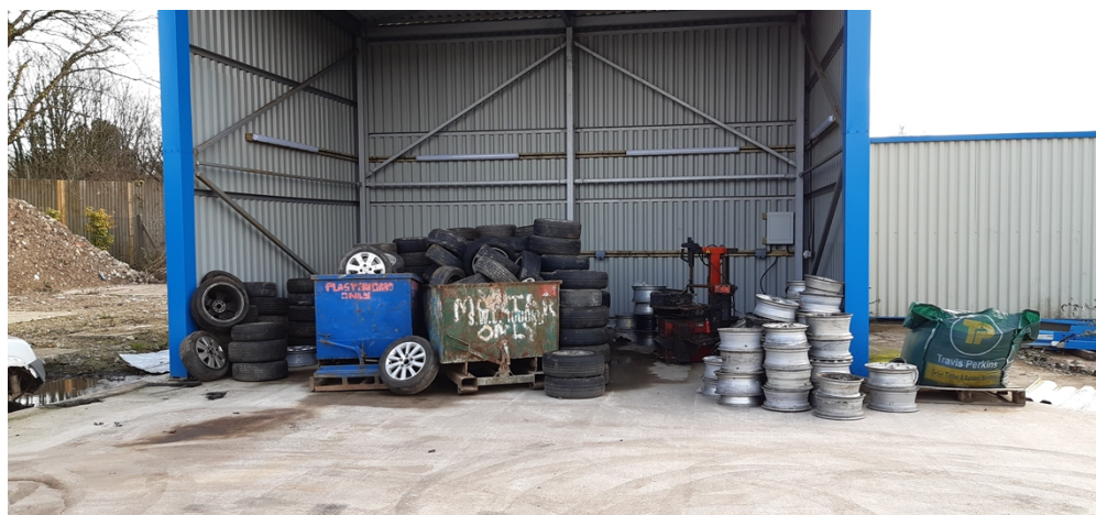
Photo 9 - Newly erected de-pollution bay at SL Recycling, Pontypool
