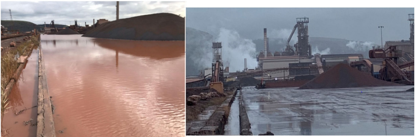
Photographs showing before and after improvements to drainage systems
