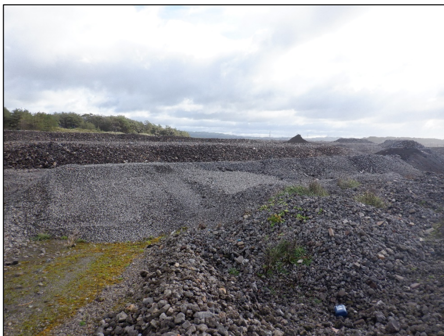
Figure 2: photograph showing the waste deposits at the hazardous landfill, covered with appropriate intermediate cover.
