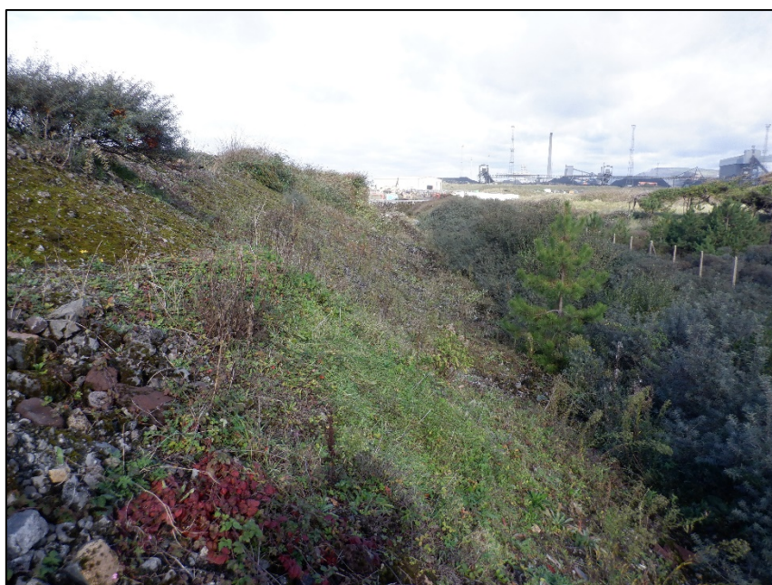
Figure 3: Photograph showing vegetation along northern flank of landfill.
