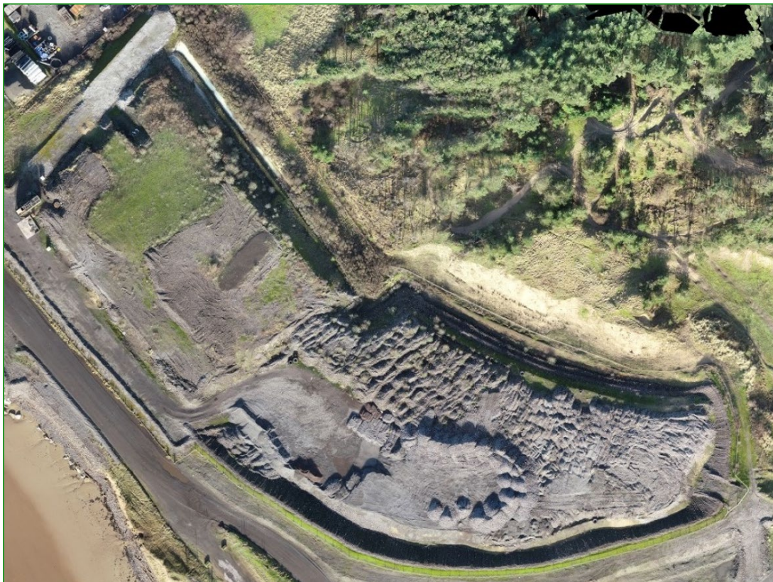
Figure 1. Aerial Photograph, showing the two operational landfill cells.
