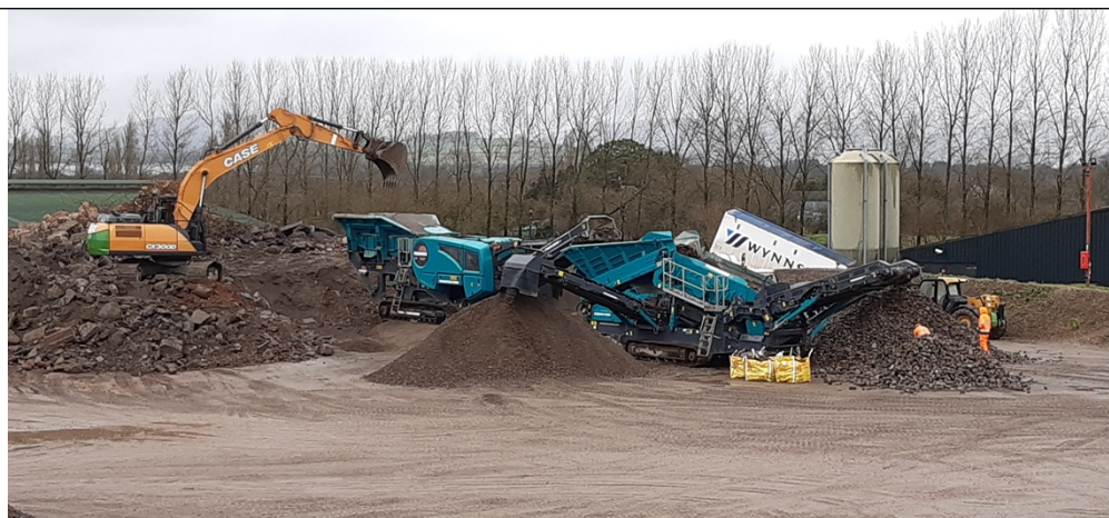
Photo 1 - On site screening operations
