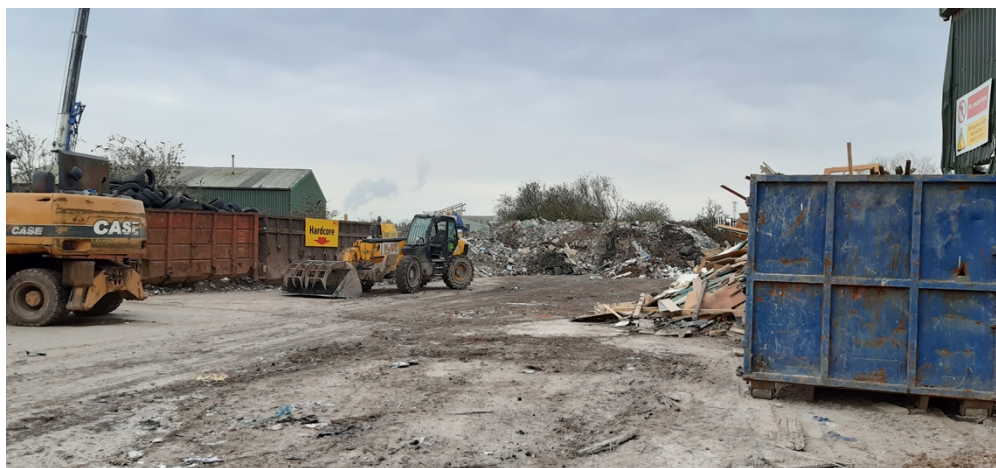
Photo 1 - General condition of site housekeeping
