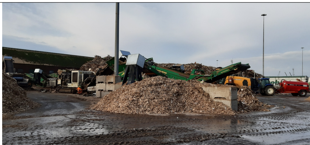
Photo 1 - General housekeeping standards were in good order on site visit
