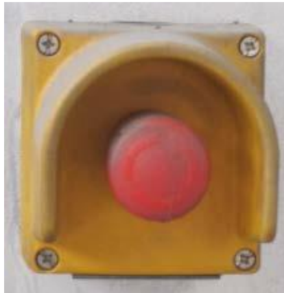
Figure 14.4-1: Emergency stop push button
