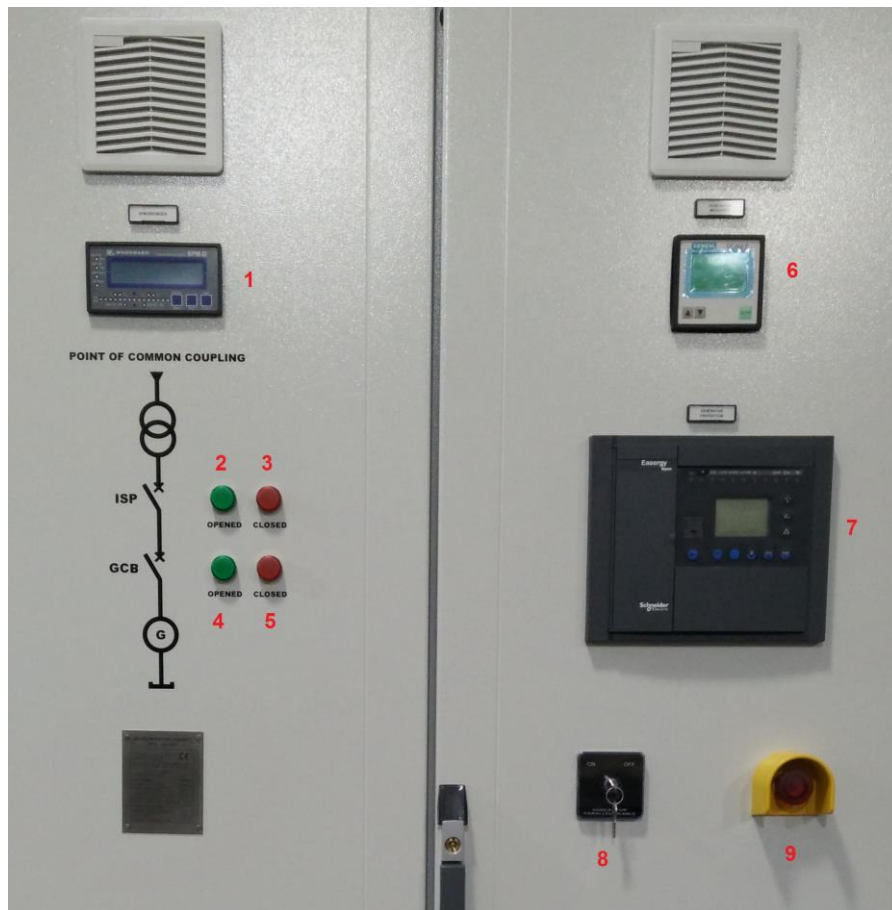
Figure 12.1-2: Synchro control panel Q0.
