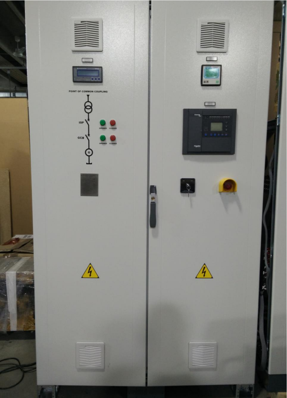
Figure 9.5-2: Q0 generator control panel.
