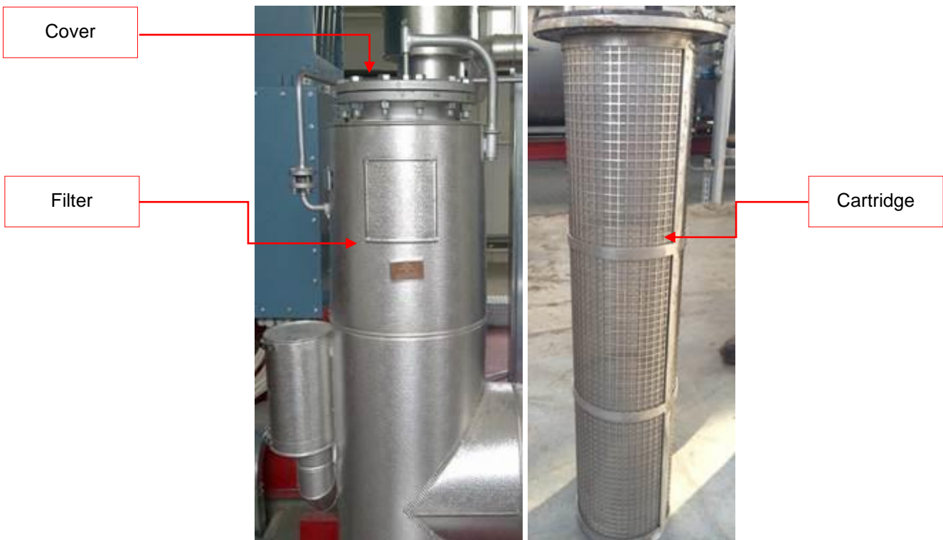
Figure 15.10-1: Feed pump filter and cartridge.
