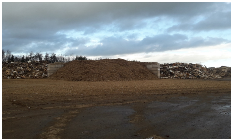
Figure 3 – stockpiled woodchip exceeding height of concrete walls during inspection on 15/12/2020
