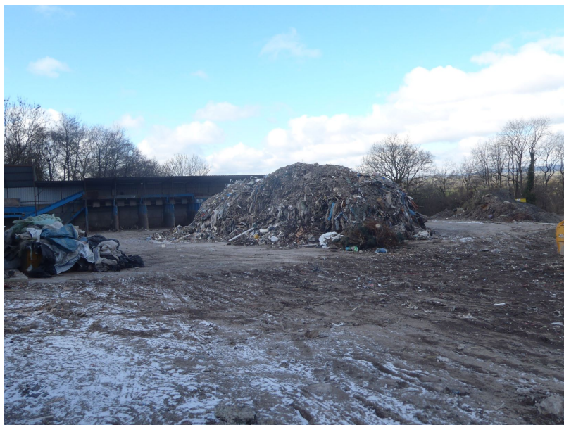
Mixed waste on impermeable pad with clear access
