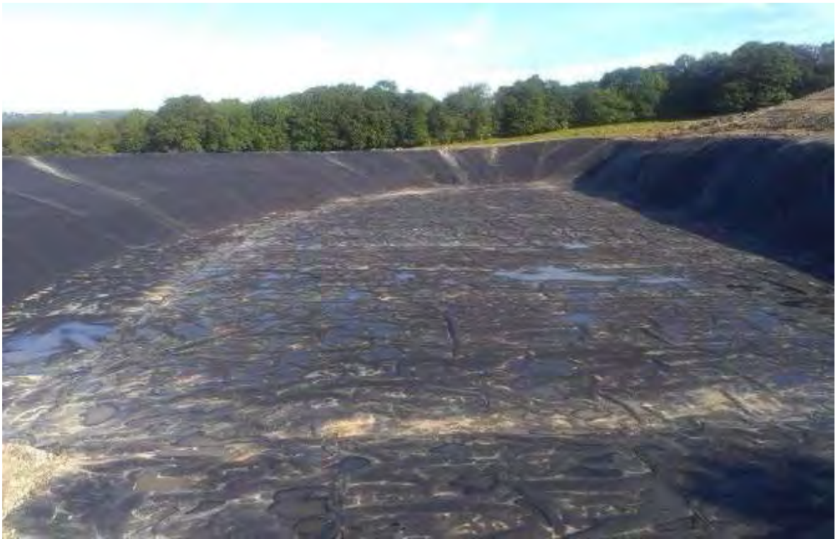
The base of the lagoon shortly after completion of the lining installation
