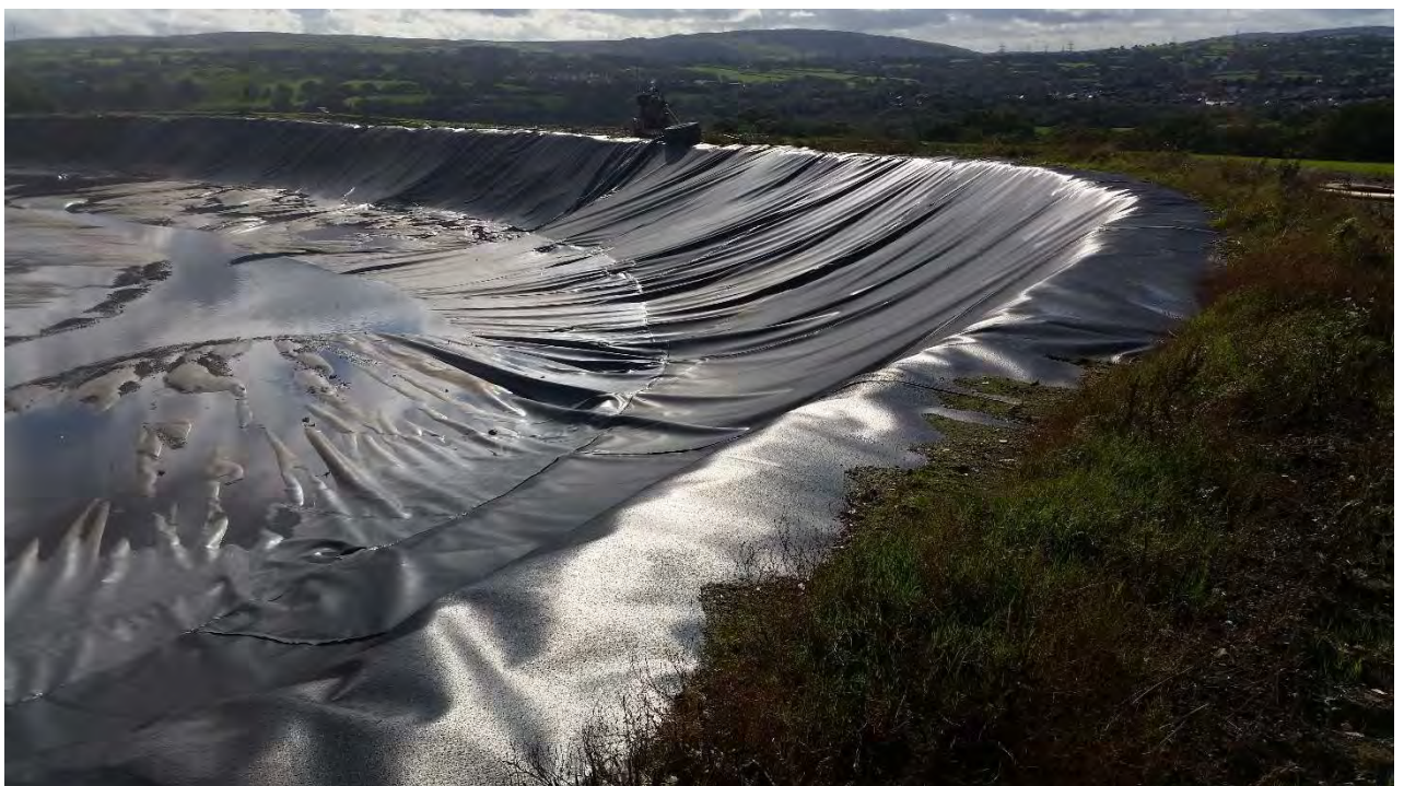
The lagoon with the floating cover installed, lagoon is partially full with puddles of naturally collected rainwater.
