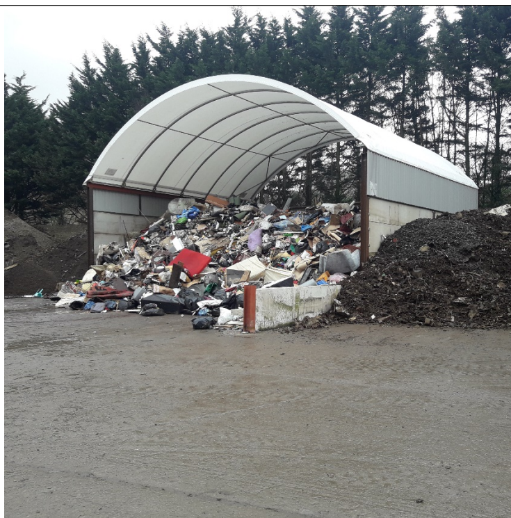
Photo One – New waste transfer station building
