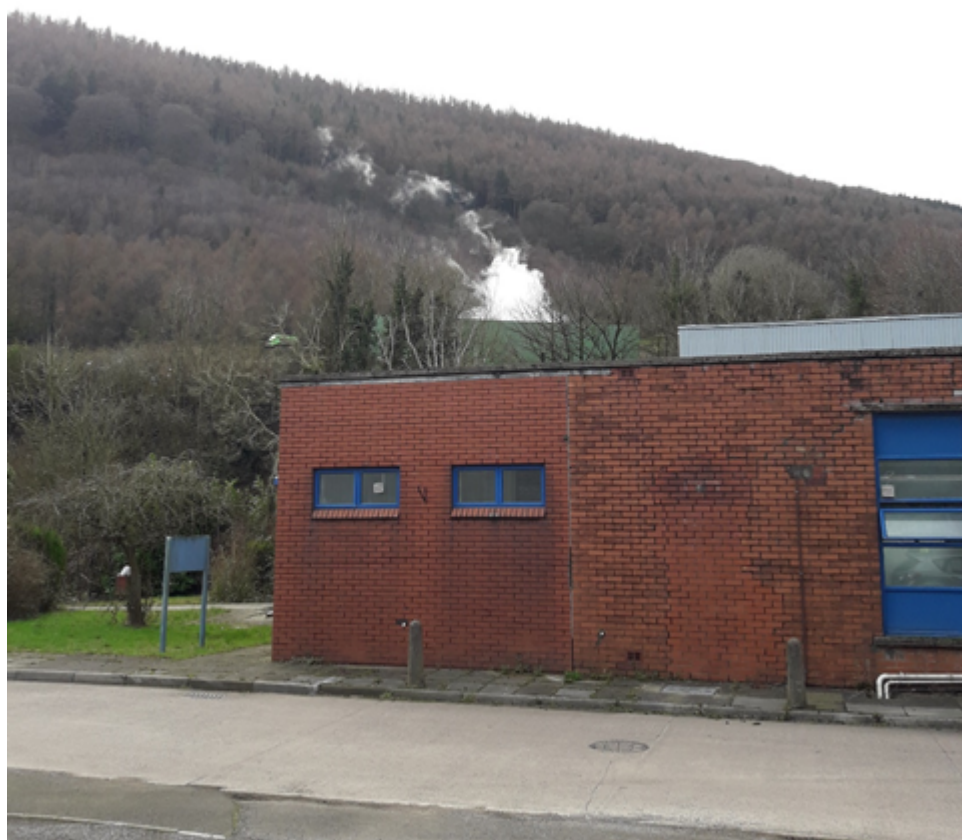
Photo Four – View of top of shredder from Chapel Farm Industrial Estate
