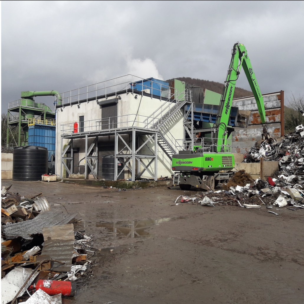
Photo Three – View of shredder, downstream plant and housing
