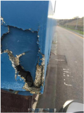
Photo A.3: Shelter 1
