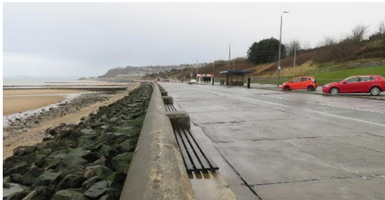
Photo 1.6: Looking East Along Promenade in Area 1
