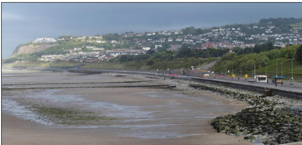
Figure 2.2: View Looking East Across the Scheme Area (proposed rock revetment to be an extension of the existing Porth Eirias revetment visible in the lower right hand corner)
