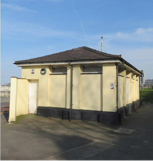
Photo A.5: Toilet block
