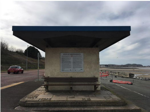
Photo A.4: Shelter 2
