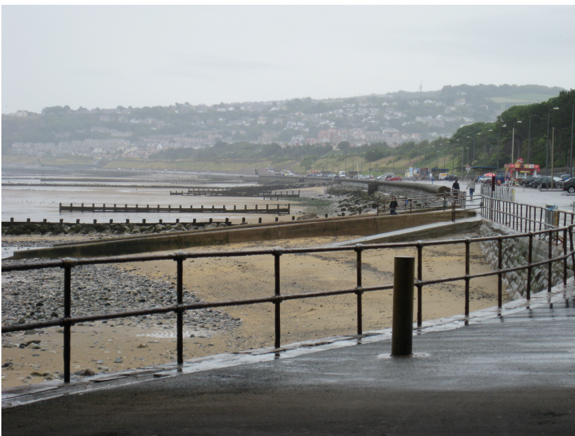
Figure 3.2: Looking east towards Old Colwyn and existing timber groynes from Victoria Pier
