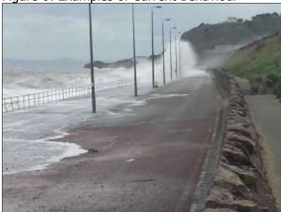
Typical overtopping on spring tide (March 2013)
