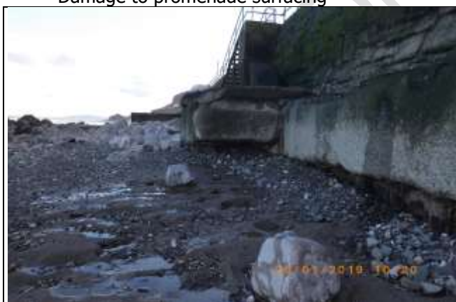
Reduction in beach levels in front of wall
