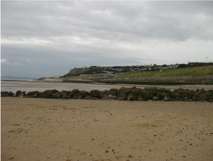
Figure 3.1: Looking eastwards towards railway embankment and existing rock groynes at Old Colwyn
