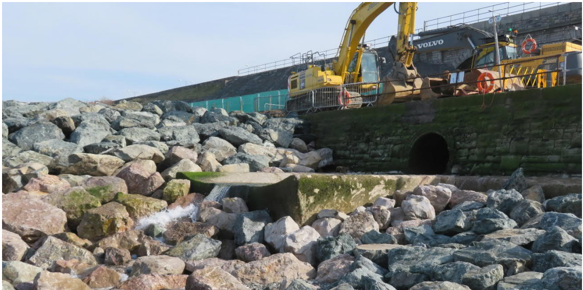
Photo 1.5: Looking North-East At Splashpoint Outfall During Revetment Construction
