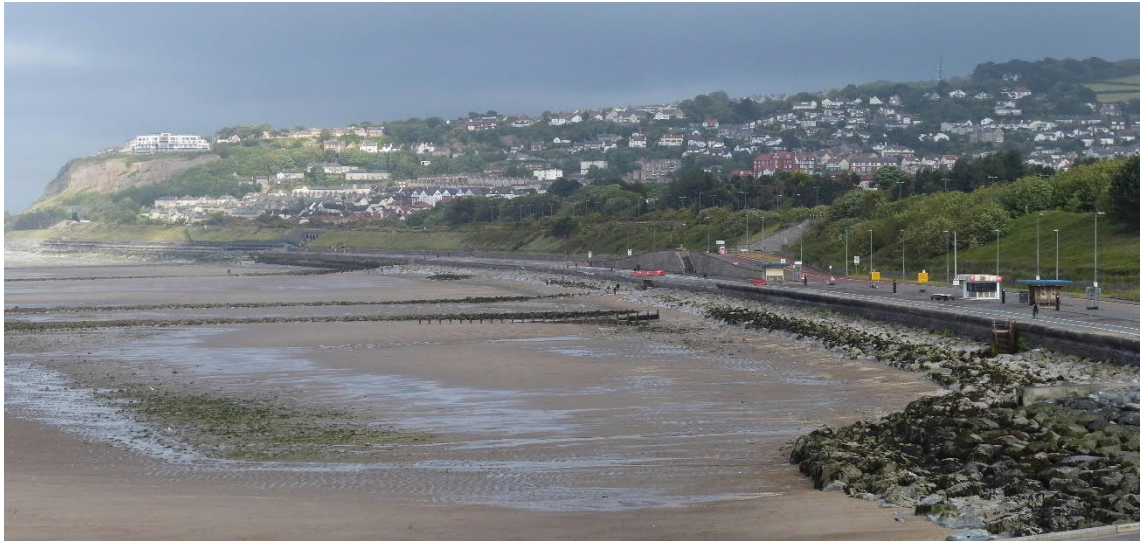
Photo 1.1: Looking East Across Scheme Area from Porth Eirias Roof Viewing Area
