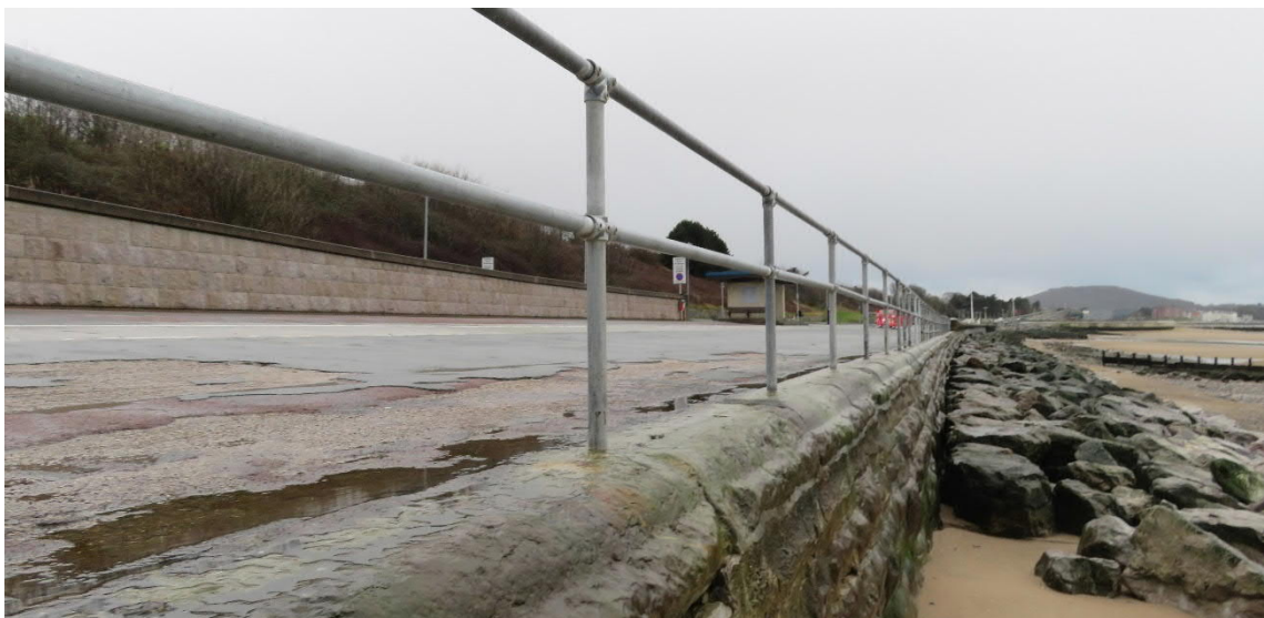
Photo 1.6: Looking West along Promenade South of Rotary Way
