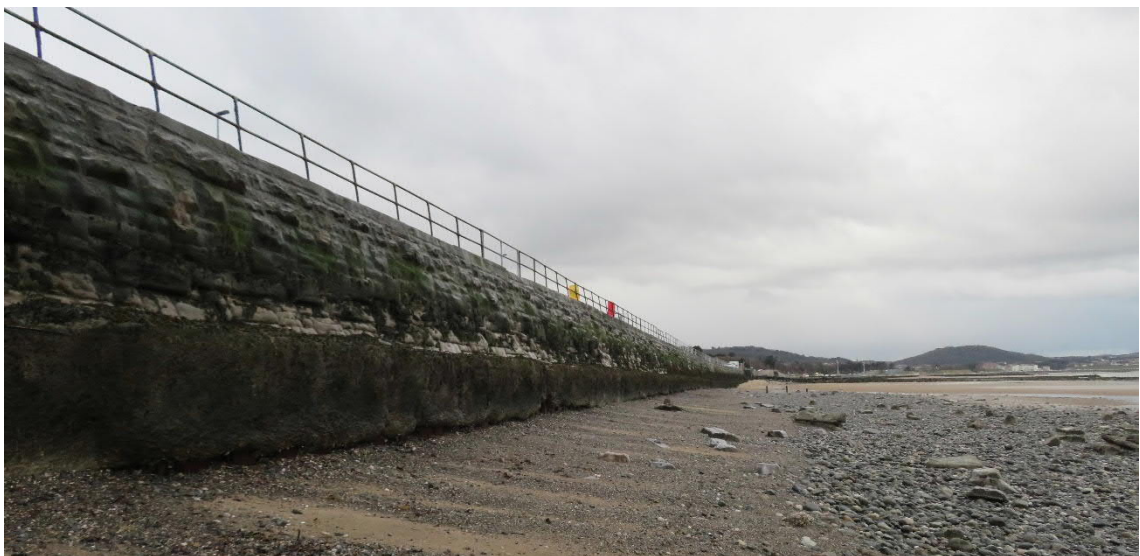
Photo 1.4: Looking West Along Sea Wall in Area 2 with Toe Protection Visible
