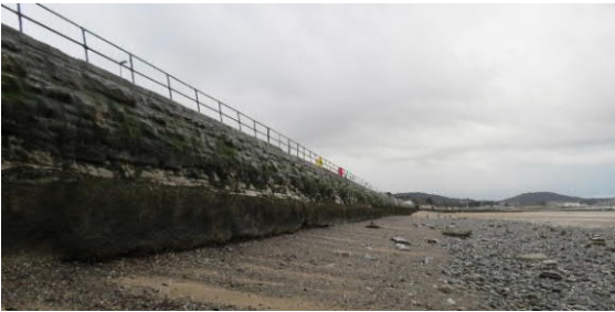
Photo 1.3: Looking West Along Sea Wall in Area 2 with Toe Protection Visible
