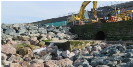
Photo 1.4: Looking North-East At Splashpoint Nant y Fynnon Outfall During Revetment Construction
