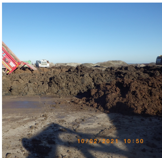
Photo of soils being tipped on site at time of visit.
