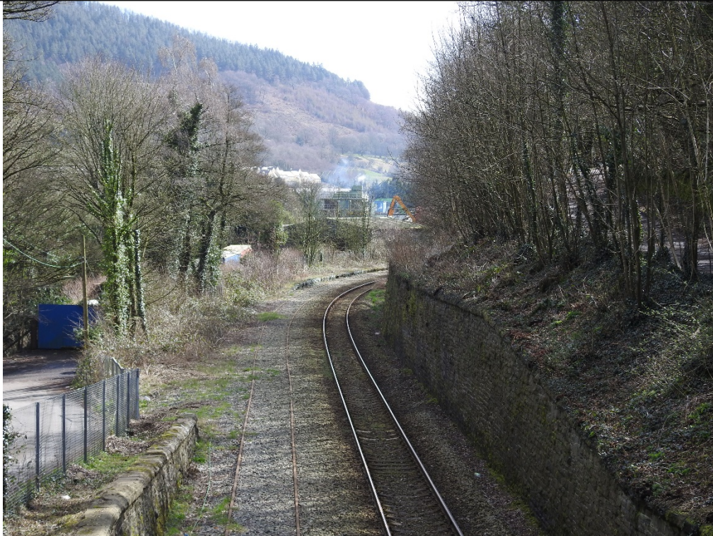
Photo One – View from bridge at end of Chapel Farm Terrace
