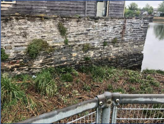
Photograph 1: Outfall location, taken from the riverbank to the west.
