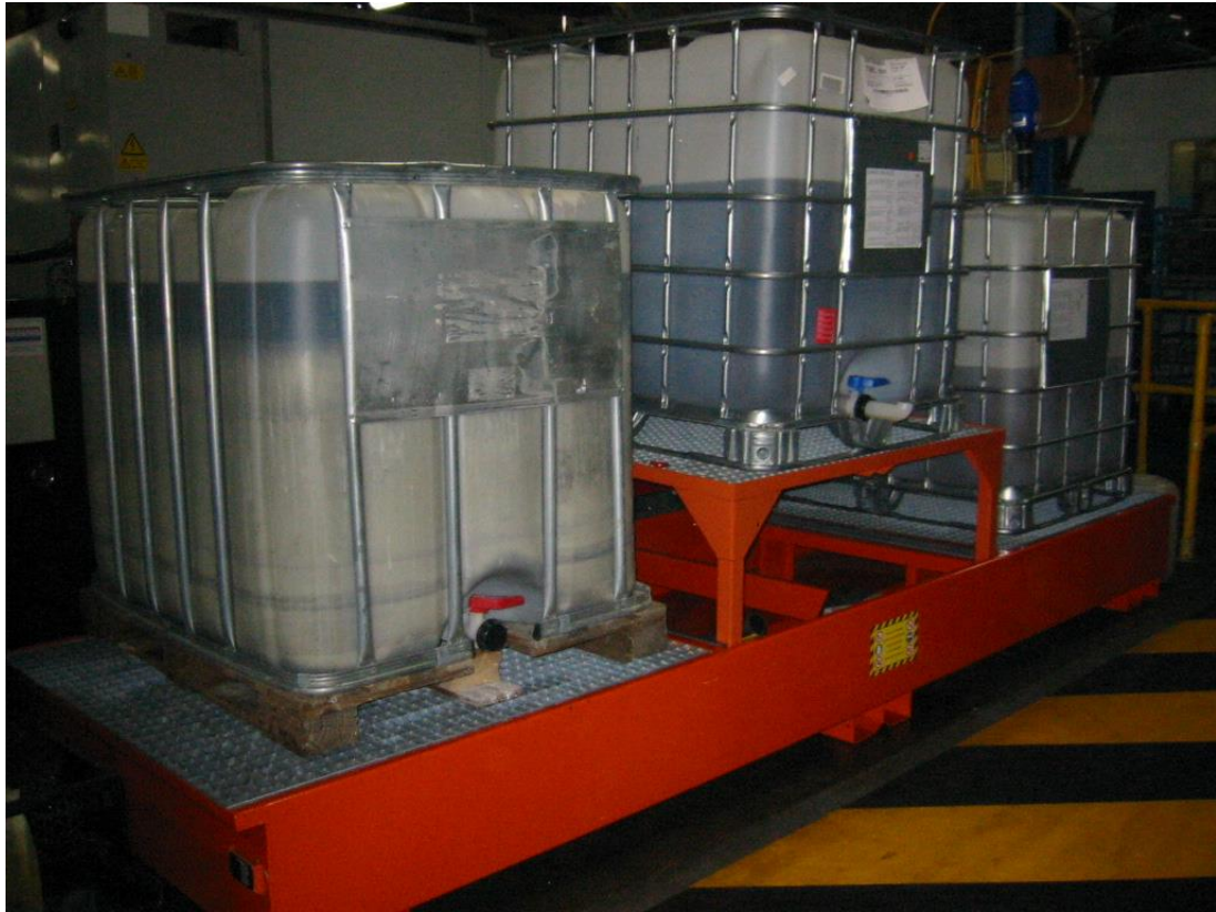
New Bund for storage of oil in Machine Shop
