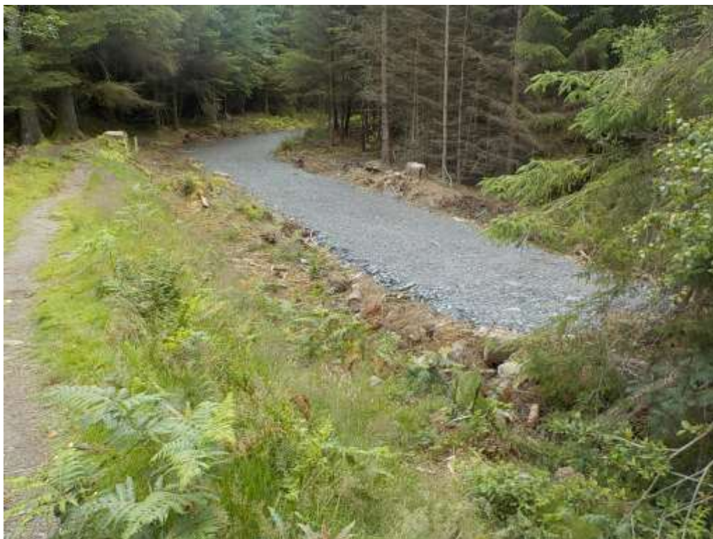
Access road installed as part of the enabling works
