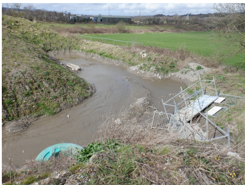
Image 1: far right hand corner of site. Drainage ditch runs to the right of image under metal walkway.
