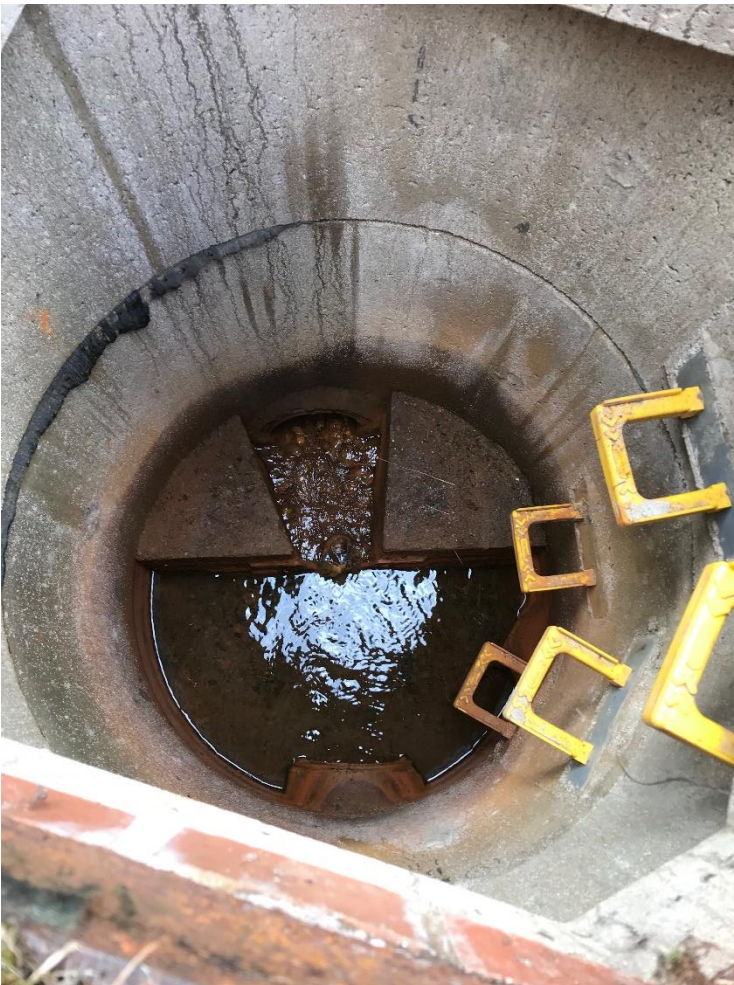
Photo B shows the confined chamber. The v-notch weir can be seen in the centre of the photo. It is thought that the weir plate is a 90 degree weir although this cannot be confirmed as access into the chamber is not permitted.
