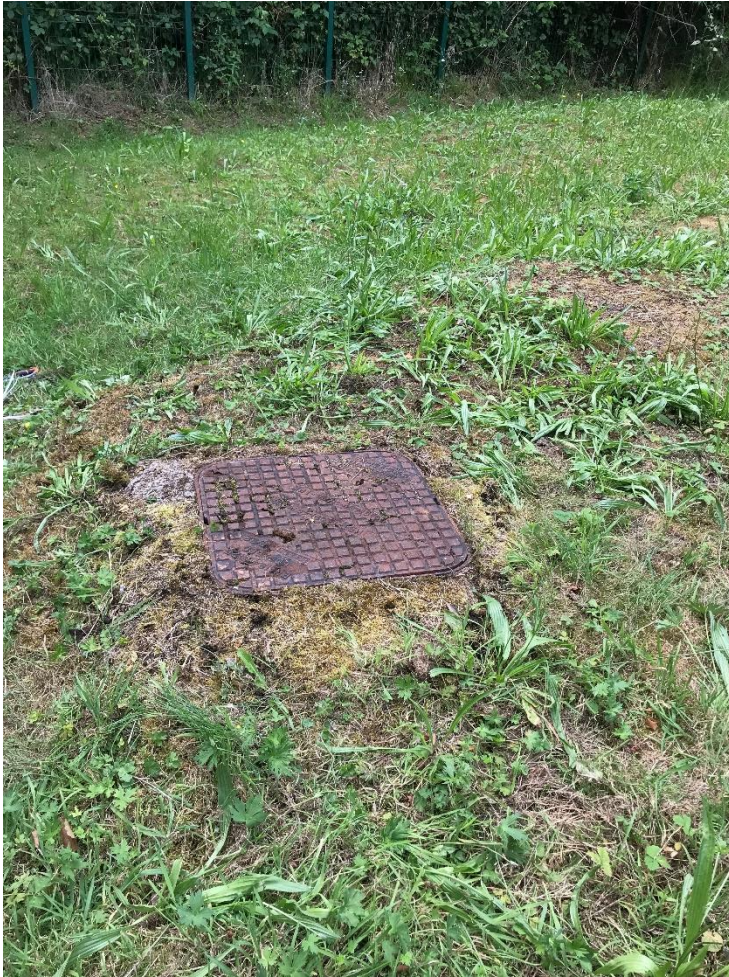
Photo A shows the access to the V-notch weir chamber.
