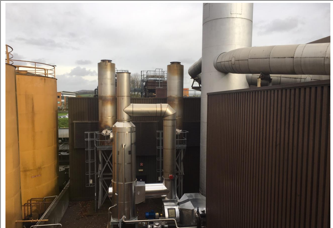
Flue Ace System- reclaim heat from emission gasses
