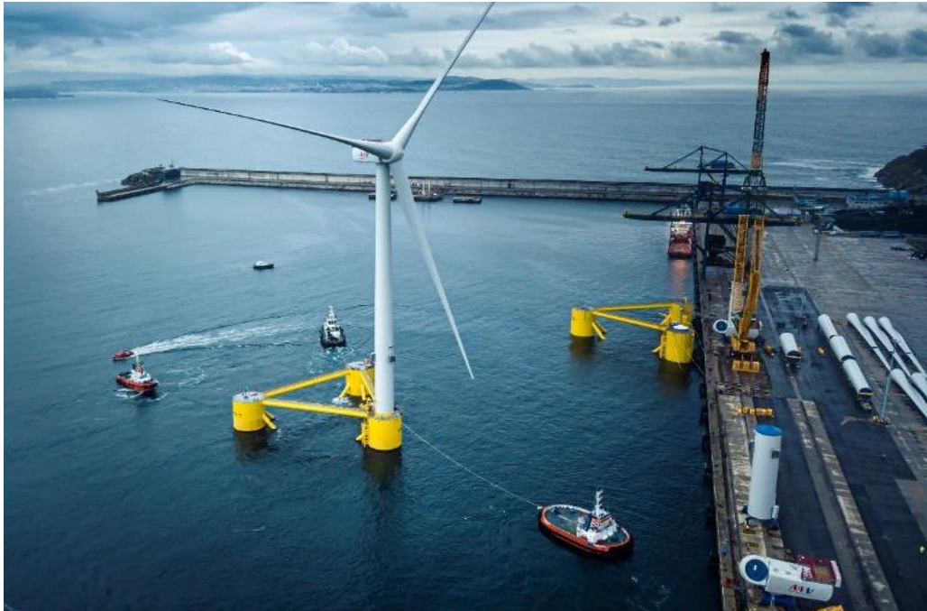
Figure 4.8 – Example of Assembly of Wind Turbine Generator onto semi-submersible WindFloat™ at quayside and towing out (Source: Photo courtesy of Principle Power. Artist: DOCK90)
