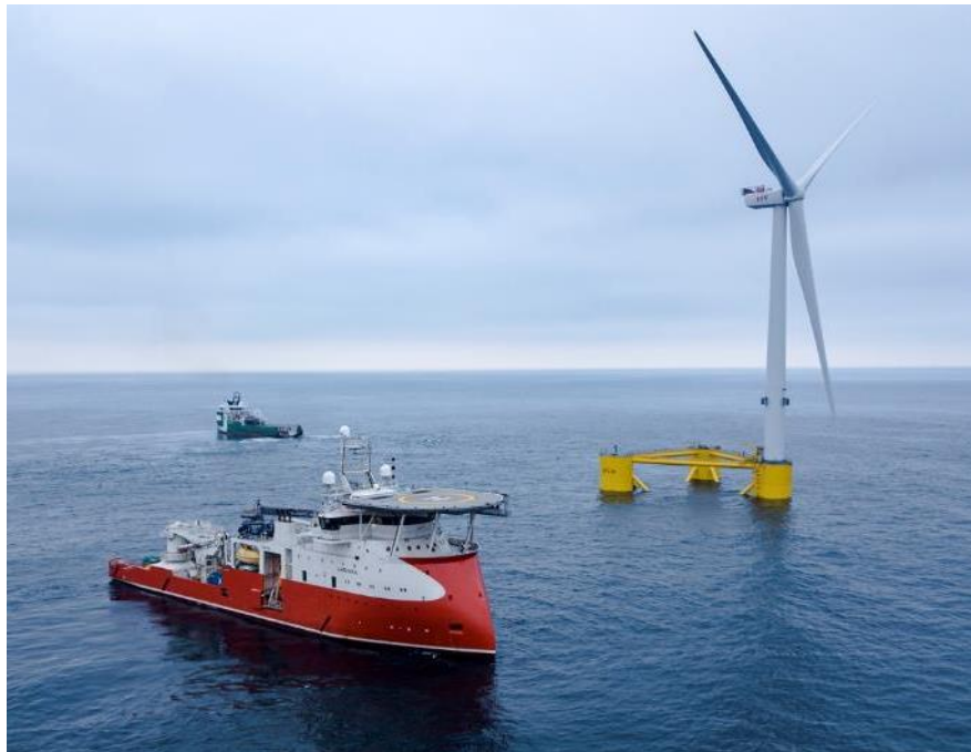
Figure 4.1 – Example Semi-Submersible Platform, WindFloat™ Atlantic Project installed in northern Portugal. (Source: Photo courtesy of Principle Power, Artist: DOCK90)
