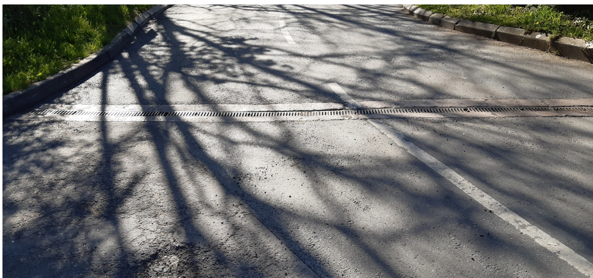
Photo 2 - Site flooring / drainage in good condition with no apparent damage/ issues
