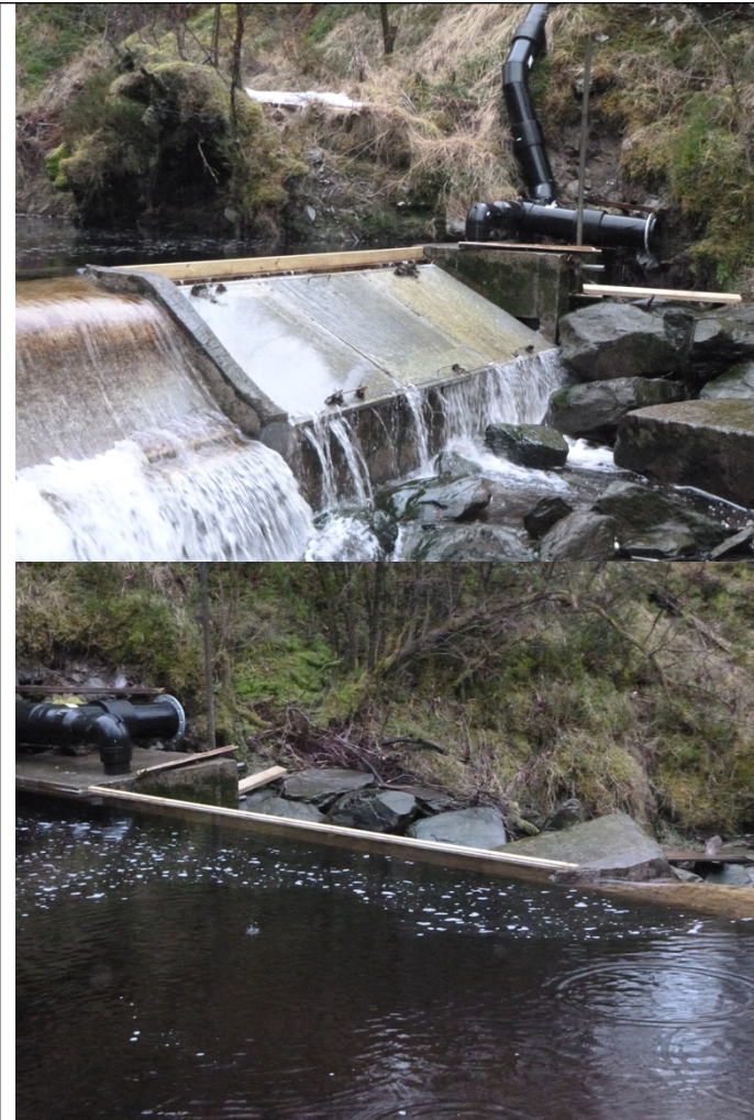
Photograph 3: Increased height of residual flow section
