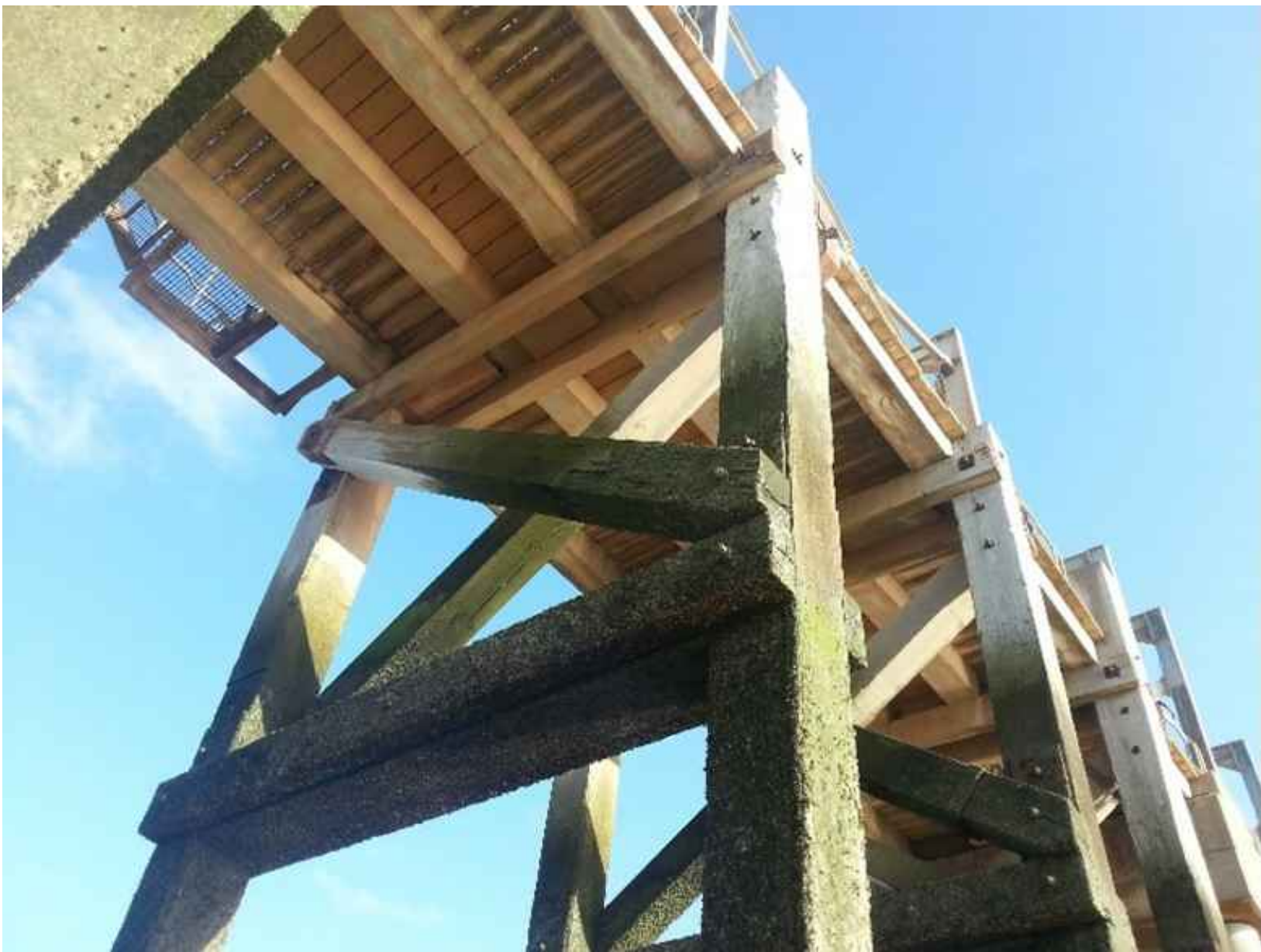
TYPICAL BAY VIEW FROM BENEATH
