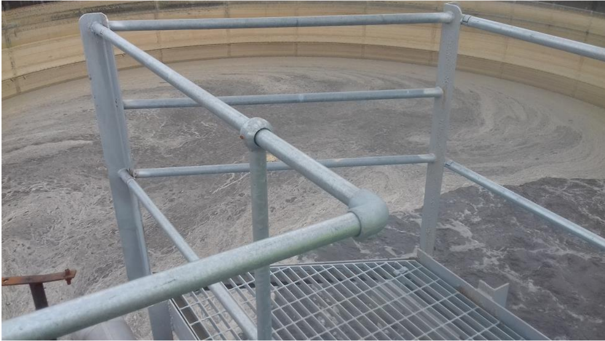
Figure 4 Balance Tank showing turbulent area under platform and foam covered area in the background
