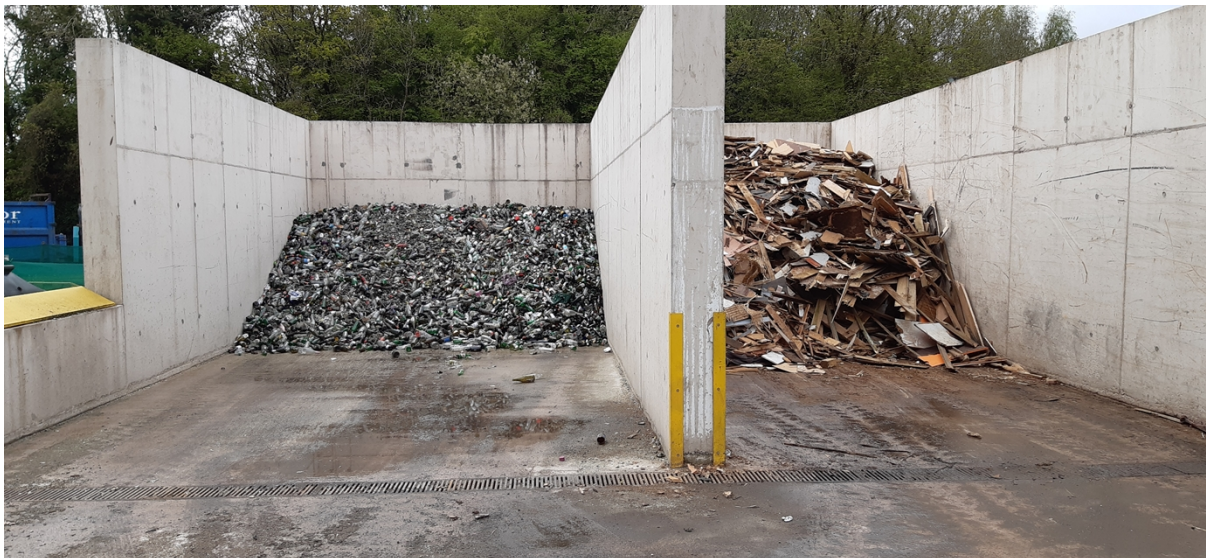
Photo 8 - Outside storage area of waste transfer station containing wood and glass bottles
