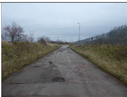
Photo. 42. Typical example of concrete roads present, with SI grassland.
