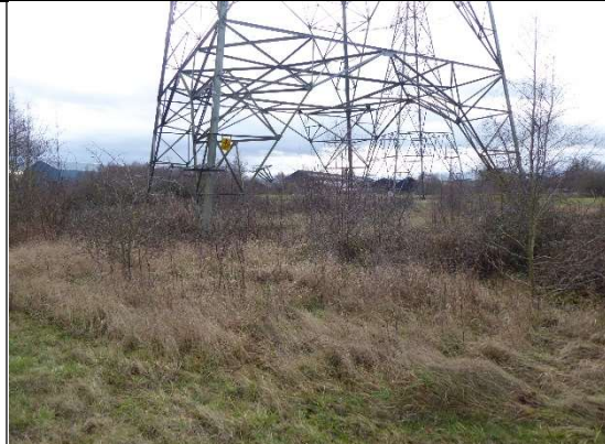
Photo. 50. Pylon at the southern end of the route.
