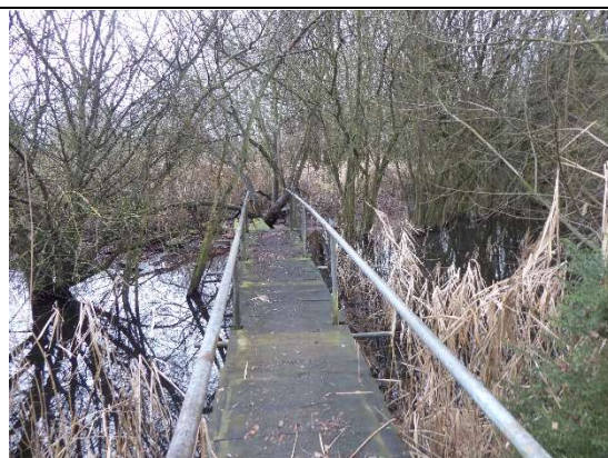
Photo. 52. Bridge over wet woodland south of the central pond.
