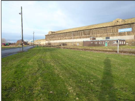
Photo. 35. Amenity Grassland where pipe route joins the North working area site
