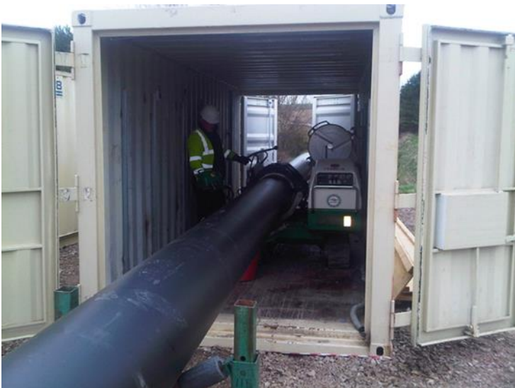
Diagram 19 : Butt Fusion Welding Shelter
