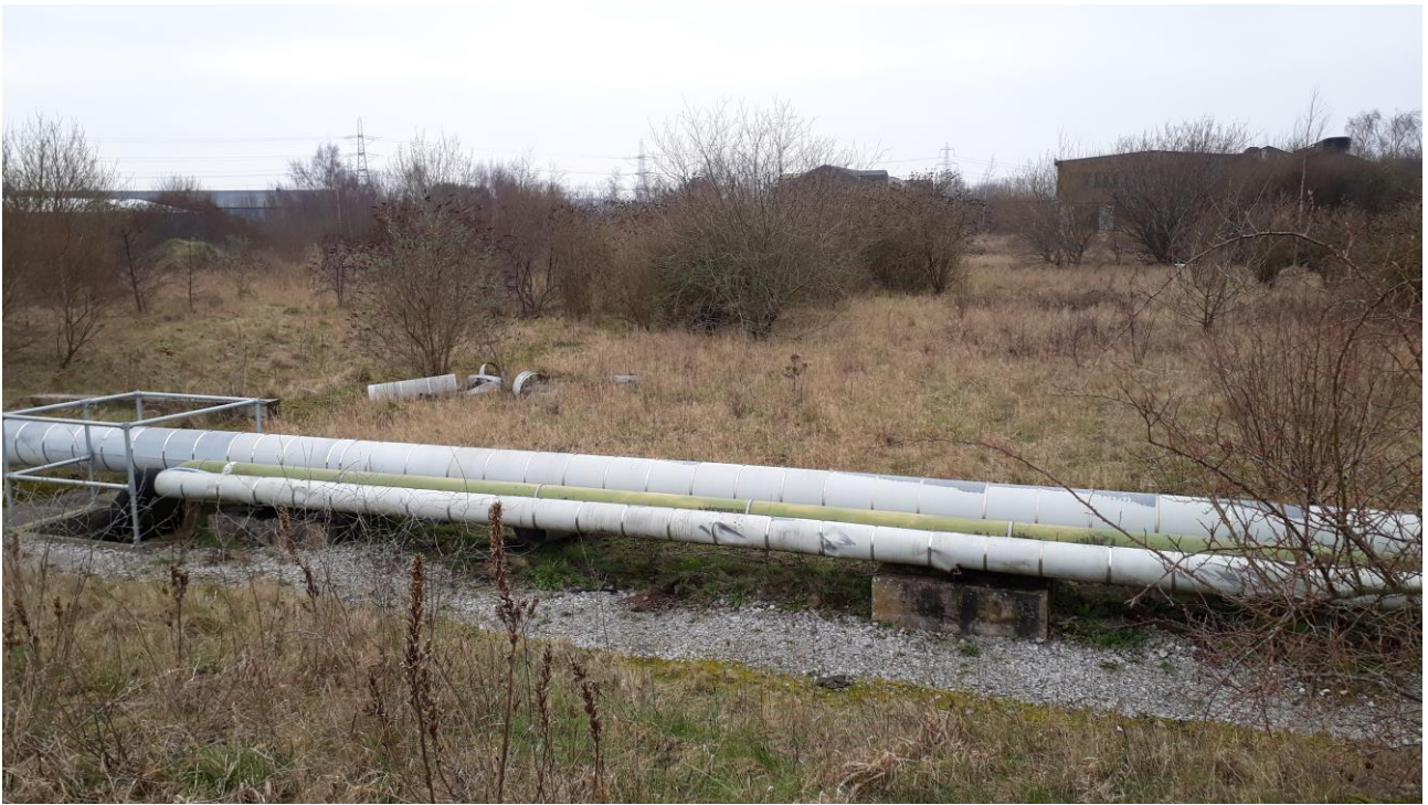
Diagram 25 : Overground Steam Pipeline on Pipeline Staging Part 1
