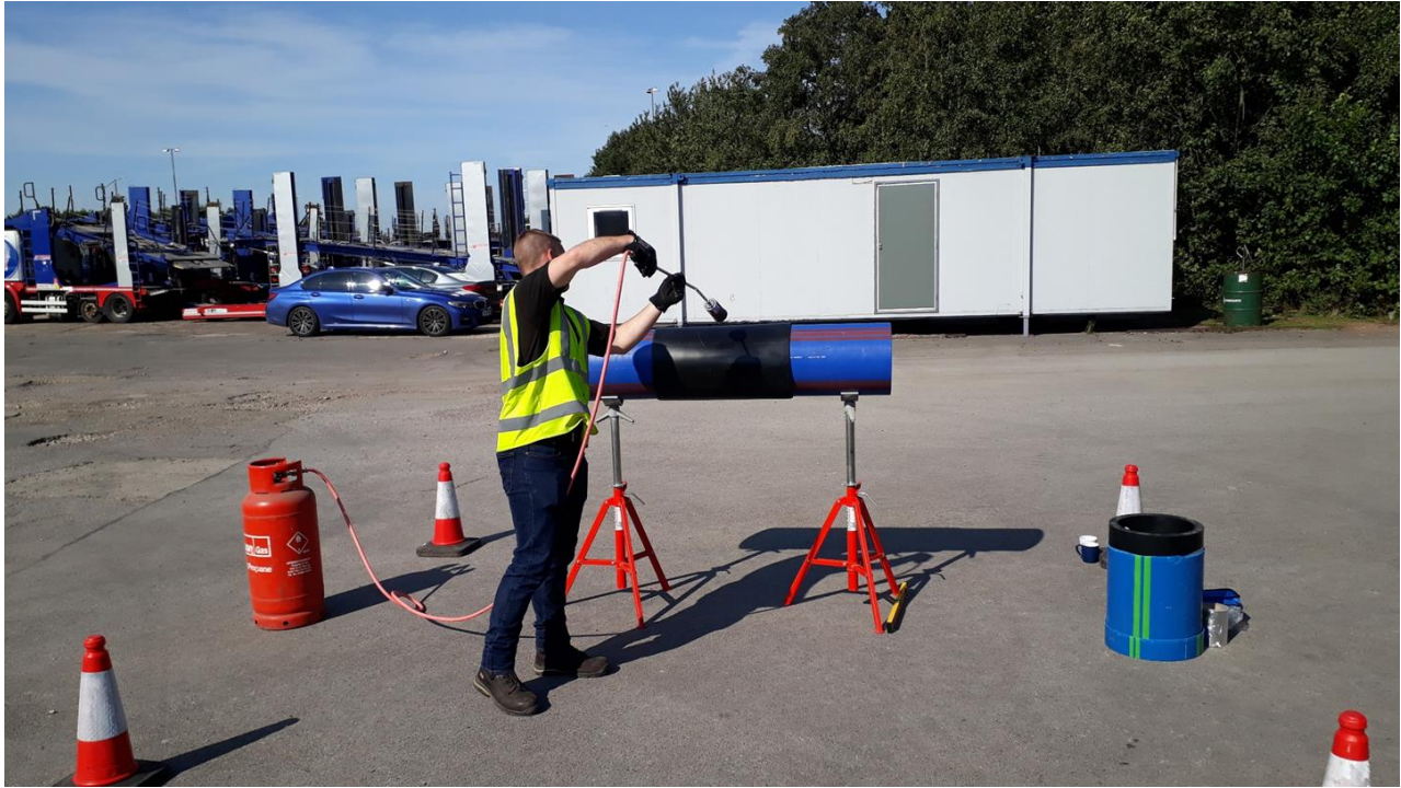
Diagram 22 : Pipeline Fabrication Stage 3 – Heat Shrink Protection
