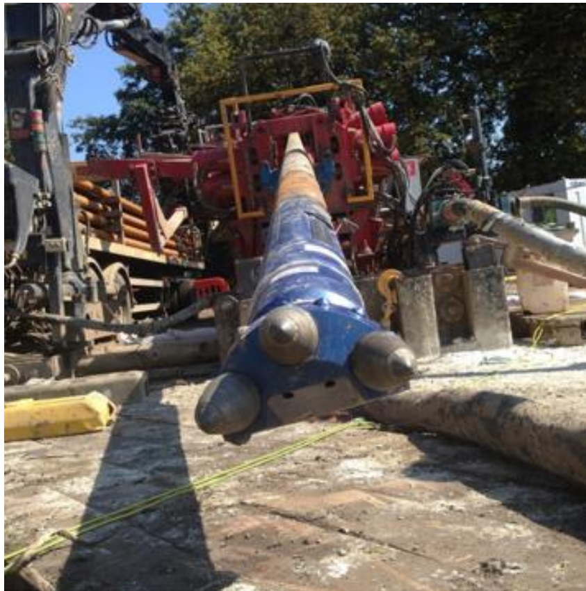
Diagram 10 : Jetting Assembly
