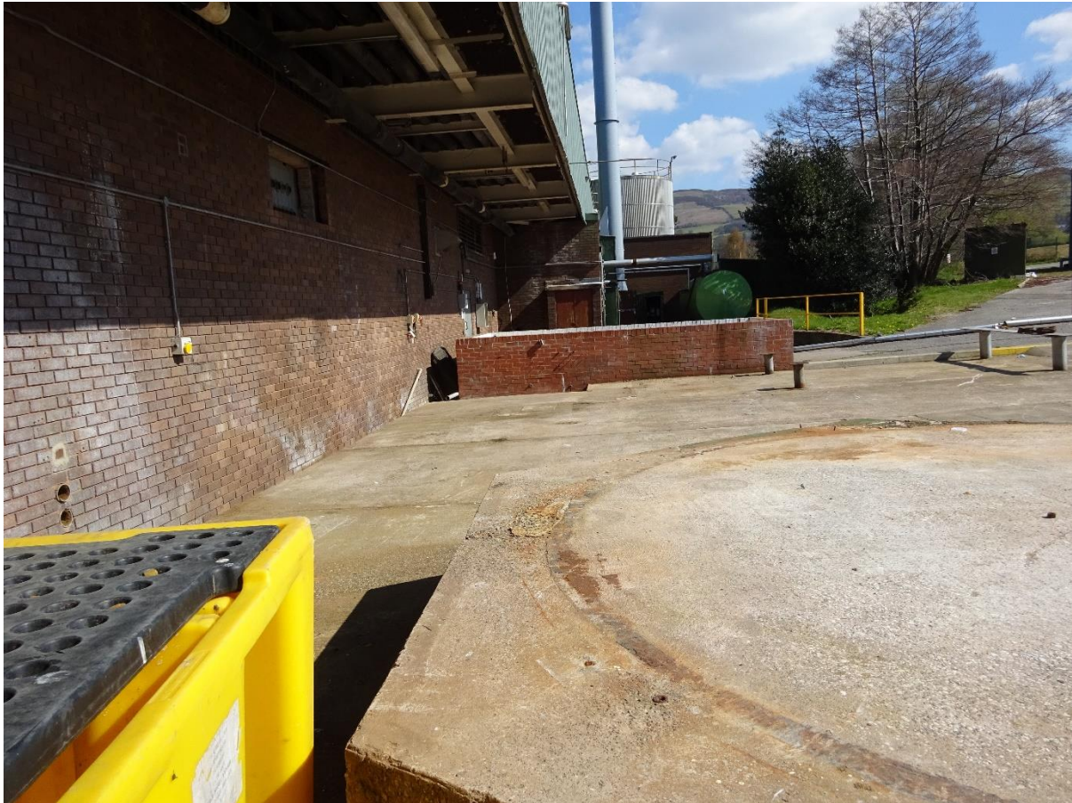
Photo 22 – Dosing chemicals bund – detached pipework breaches the wall on the left side
