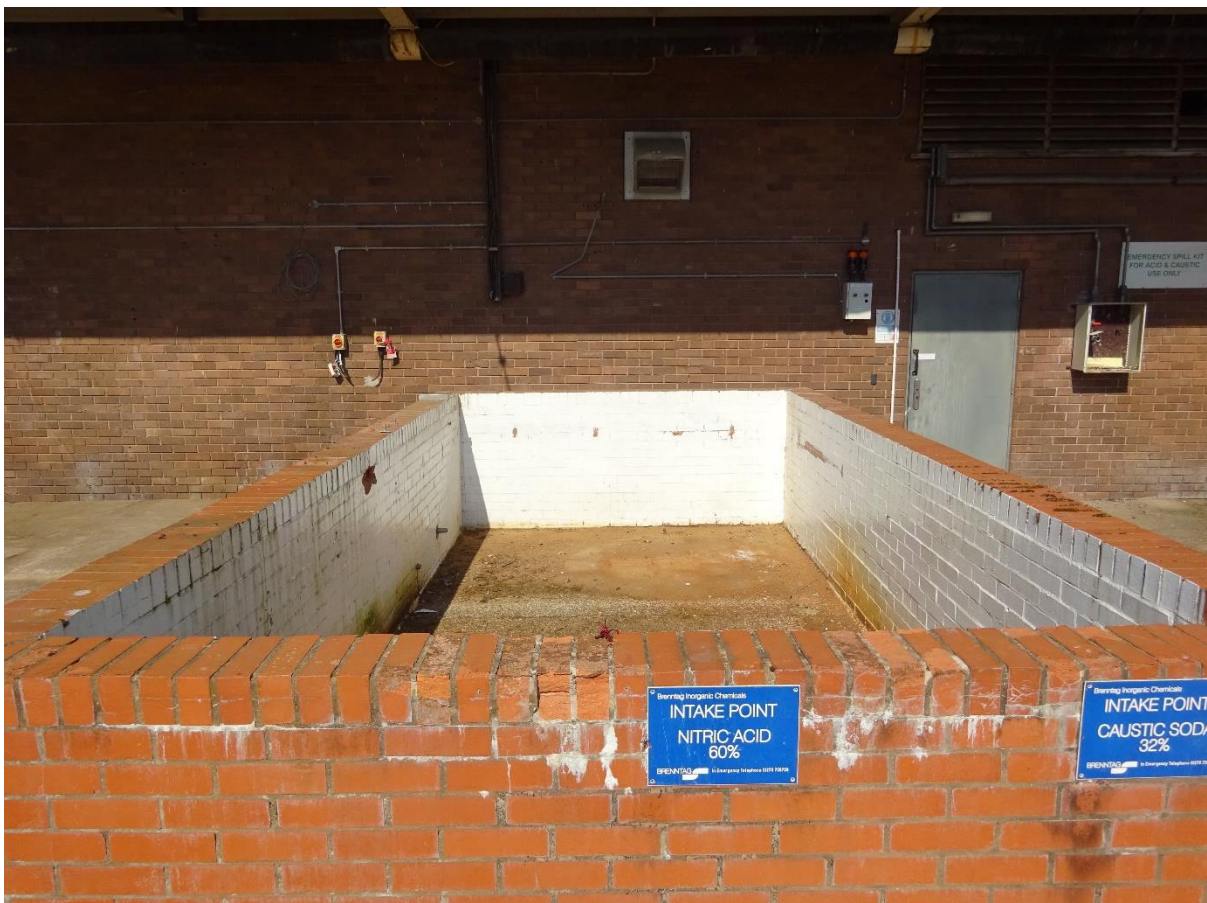
Photo 22 – Dosing chemicals bund – detached pipework breaches the wall on the left side
