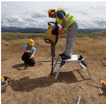
Figure 4: Operating the percussion corer
