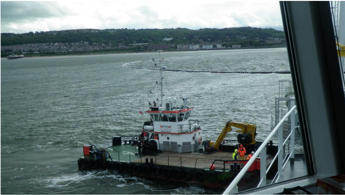
Photo 2.2: Beach recharge works during previous phase – view from TSHD of the floating pipeline
