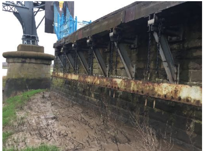
River facing wall of east bank deck
