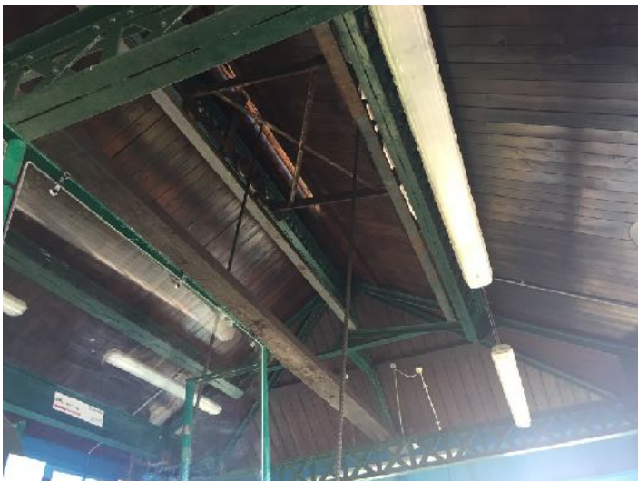
Interior view of the winch house
