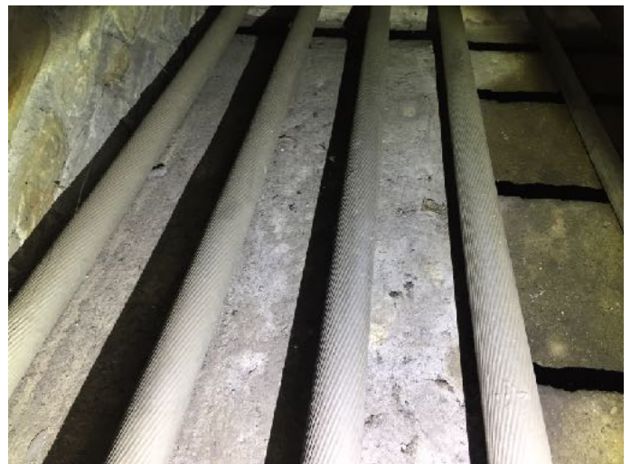
View of concrete floor
