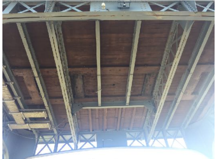
View underneath the winch house
