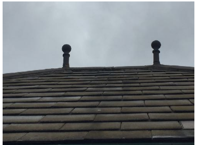
View of visitor centre roof with slight raised tiles
