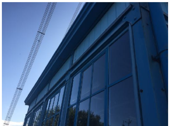
Winch House east elevation
