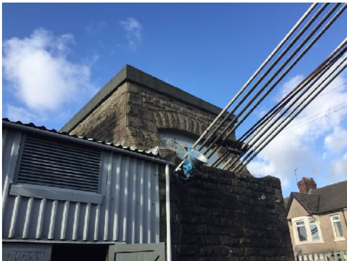
West Bank anchorage house
