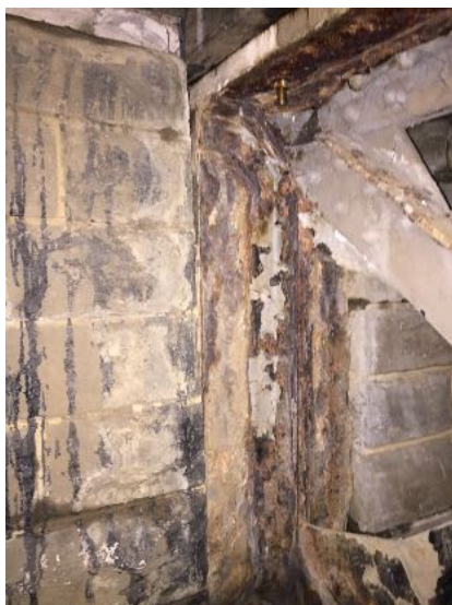
View of wall that deck metal work sits in
