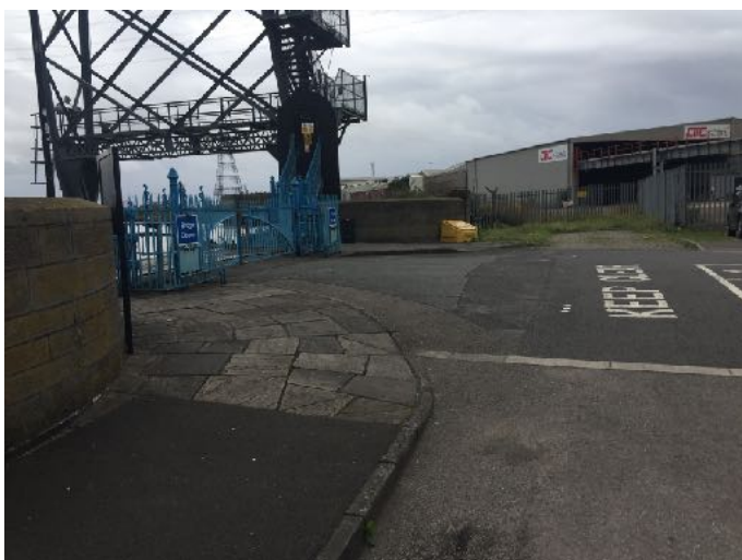
View of bridge loading western bank
