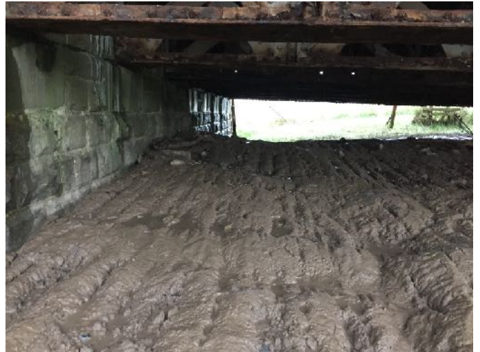
View underneath east bank deck
