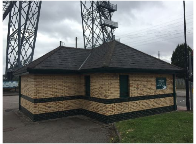
View of visitor centre roof with slight raised tiles
