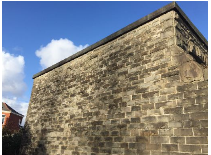
West Bank anchorage house
