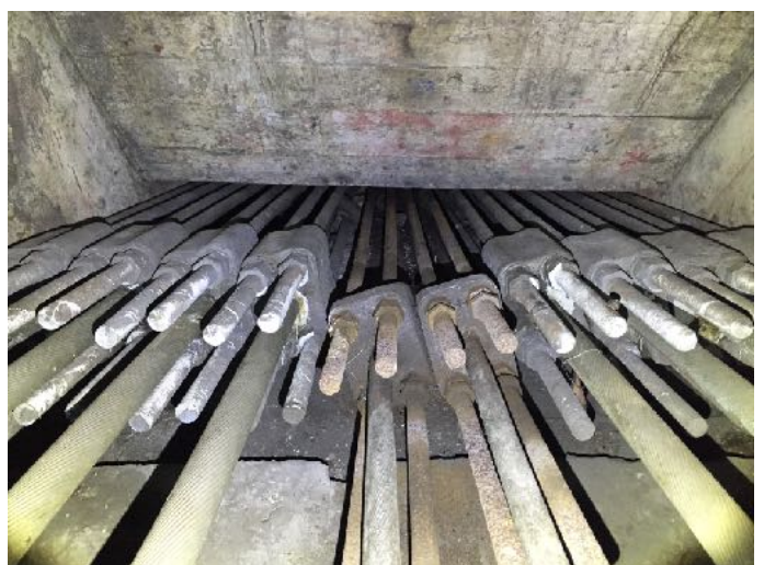
View of cables sunken into the ground
