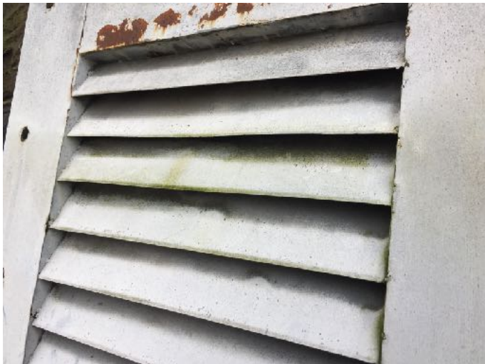
View of grilled entrance cover
