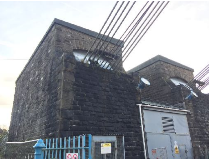
East bank anchorage house
