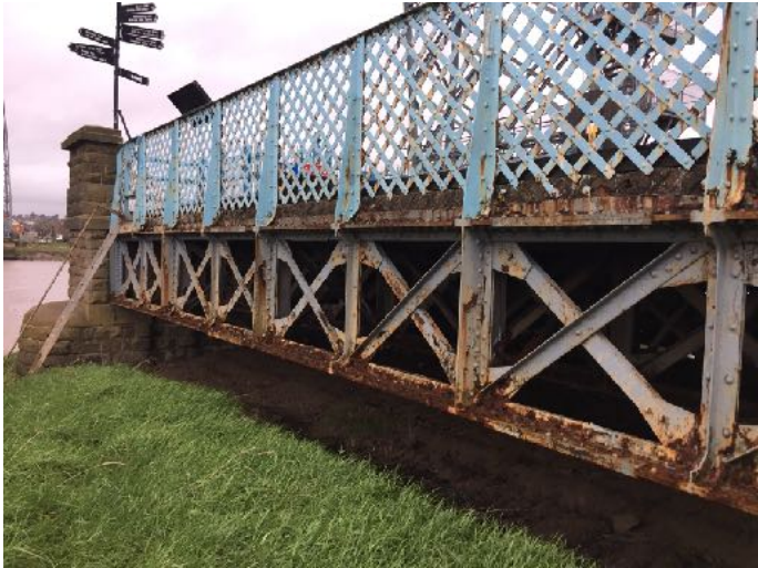
Side view of east bank deck
