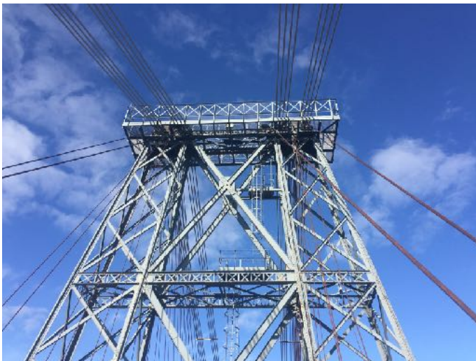
View of bridge tower
