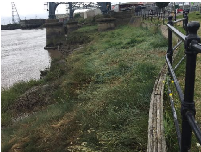
View of retaining wall and bridge footings
