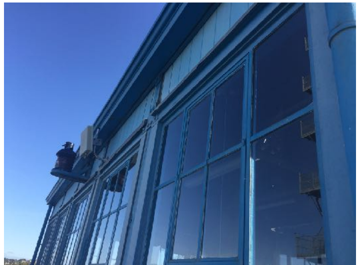
Winch House south elevation
