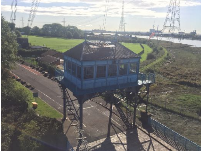
View of Winch House
