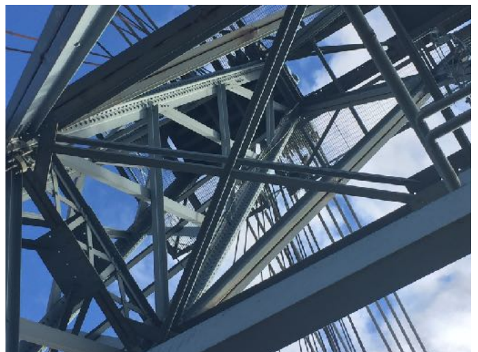
View of tight metal work
