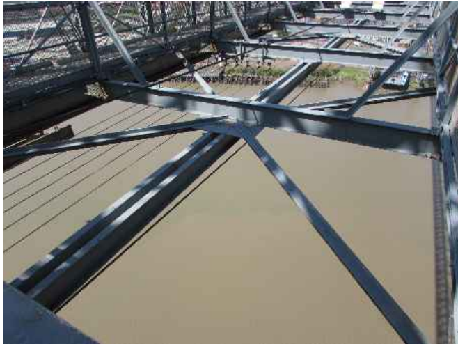
Main Boom Traveller Steelwork General overview of the Main boom steelwork.
