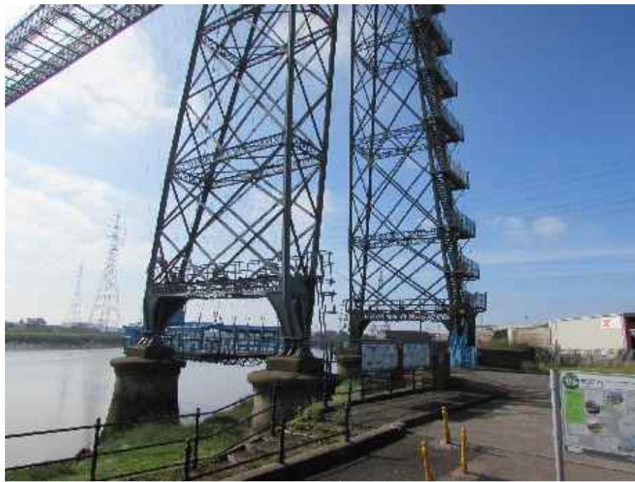
West Pylon General view Photo taken: 24-07-2019
