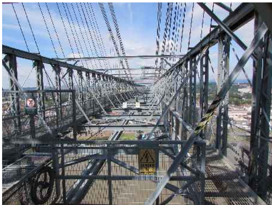
Main Boom General view Photo taken: 24-07-2019
