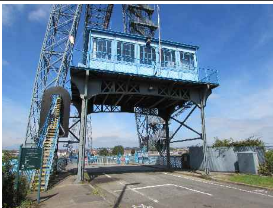
Motor House General view Photo taken: 24-07-2019
