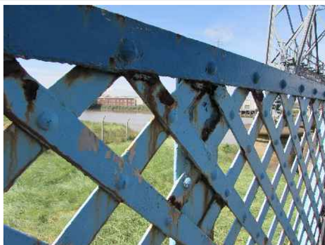
Eastern Approach Topside Lattice
