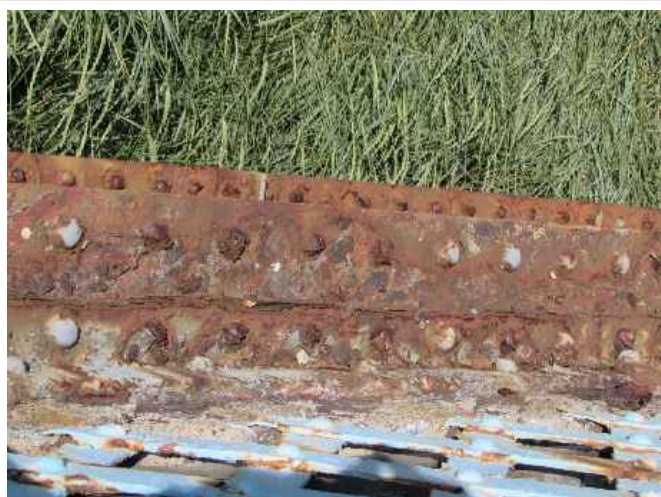
Eastern Approach Underside
