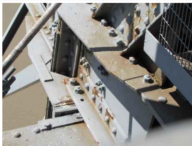
Main Boom Primary Steelwork
