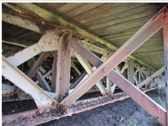
Eastern Approach Underside
