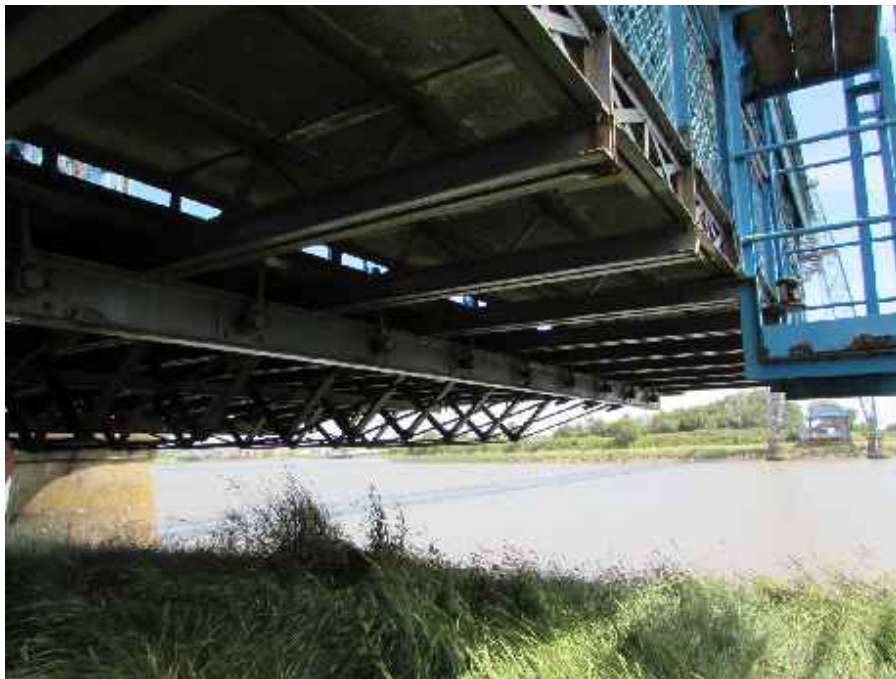
Gondola Underside General view Photo taken: 24-07-2019
