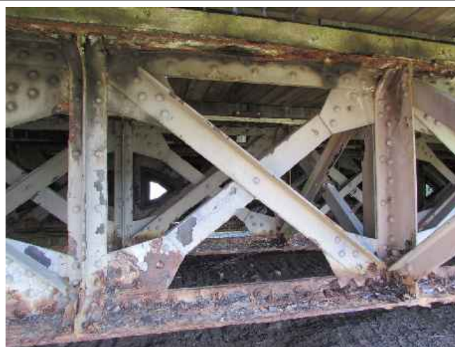
Eastern Approach Underside
