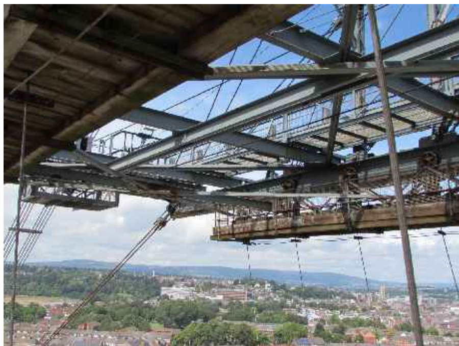
Main Boom General view Photo taken: 24-07-2019
