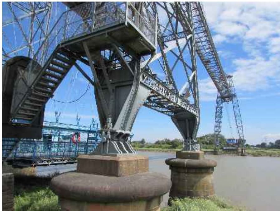
West Pylon Photo taken: 24-07-2019
