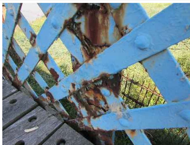
Eastern Approach Topside Lattice
