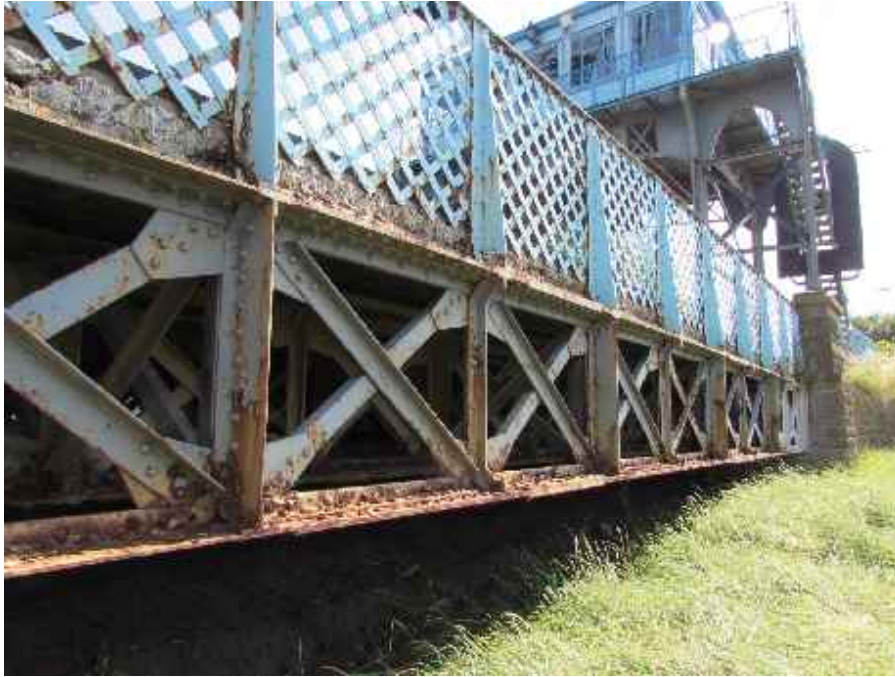
Eastern Approach Underside Photo taken: 24-07-2019
