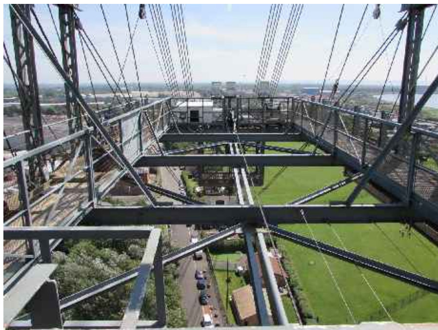
Main Boom General view Photo taken: 24-07-2019
