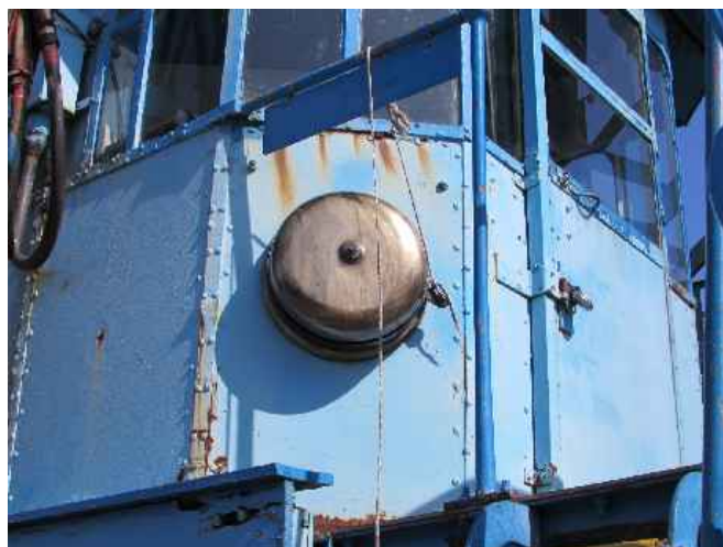
Gondola Topside General overview of Gondola drivers cabin.
