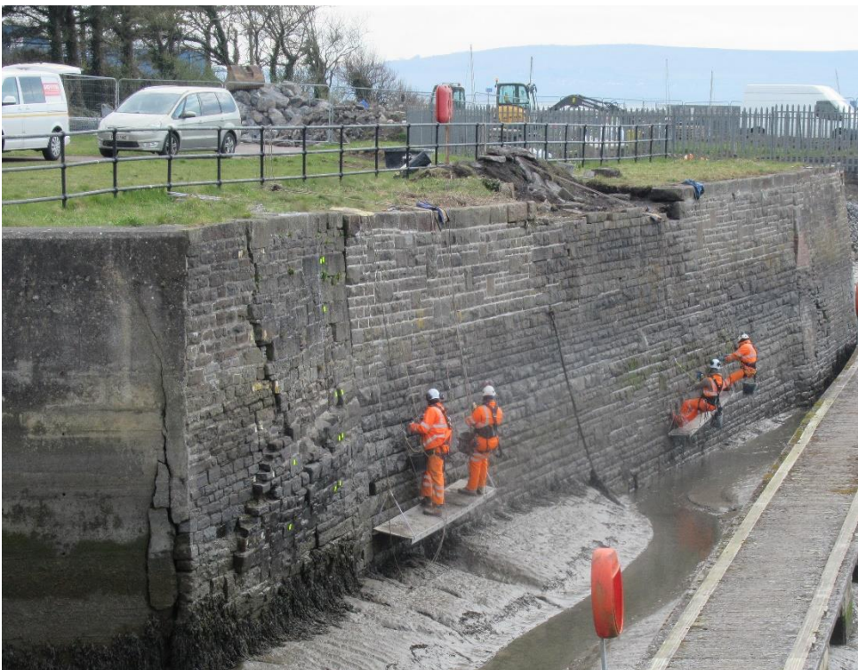
Photo 10 - Repointing and wall repairs by rope access
