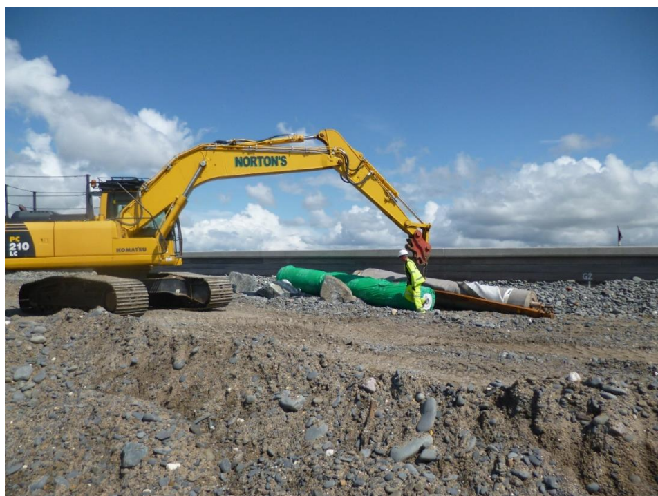
Photo 2 – Tracked excavator placing geotextile
