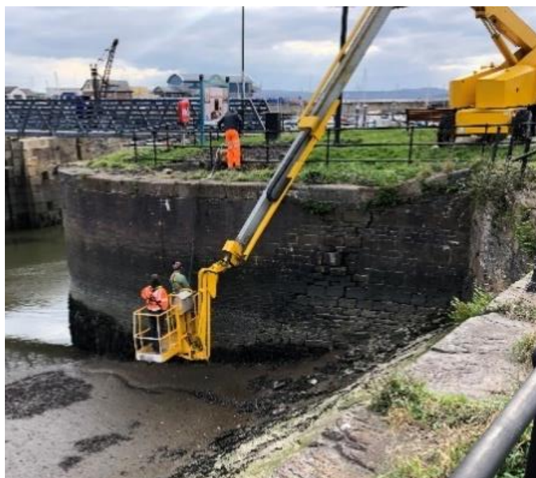
Photo 8 - Negative Mobile Elevated Working Platforms (MEWP's) to repair walls from above high water
