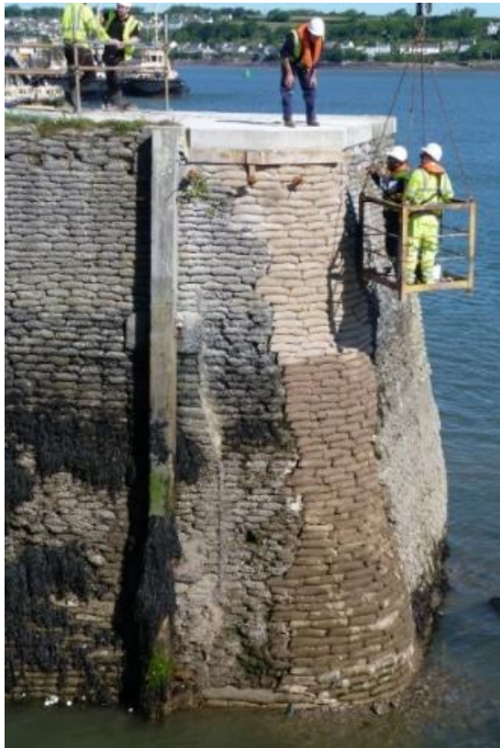
Photo 10 - Repointing and wall repairs by rope access
