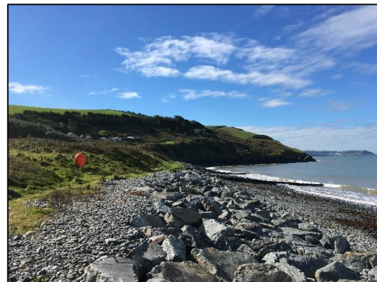
Figure 1-4 Rock Revetment along South Beach
