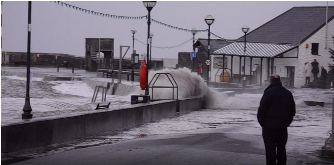
Figure 1-2 Flooding along Quay Parade
