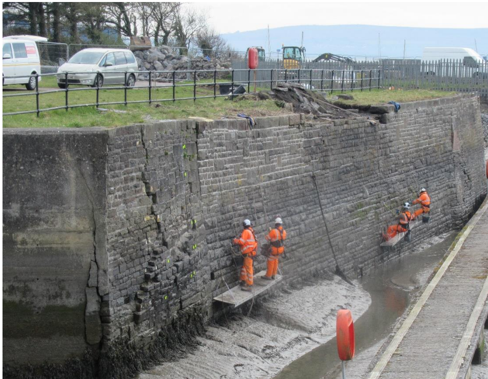
Figure 1-11 - Repointing and Wall Repairs by Rope Access
