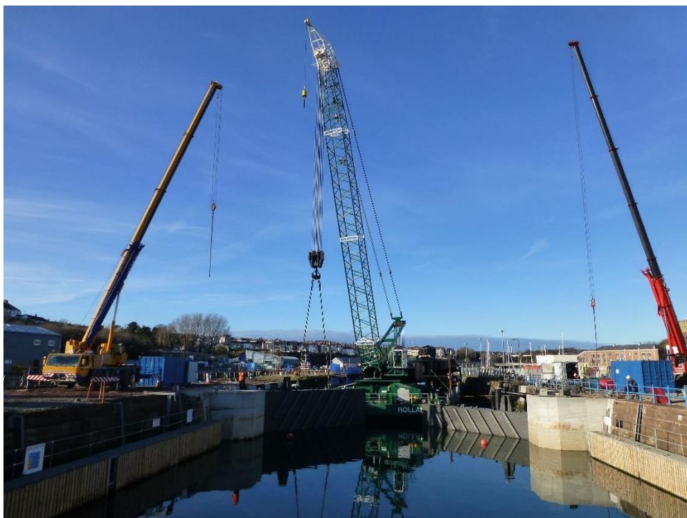
Figure 1-13 Barge, Crane and Gate at Milford Marina
