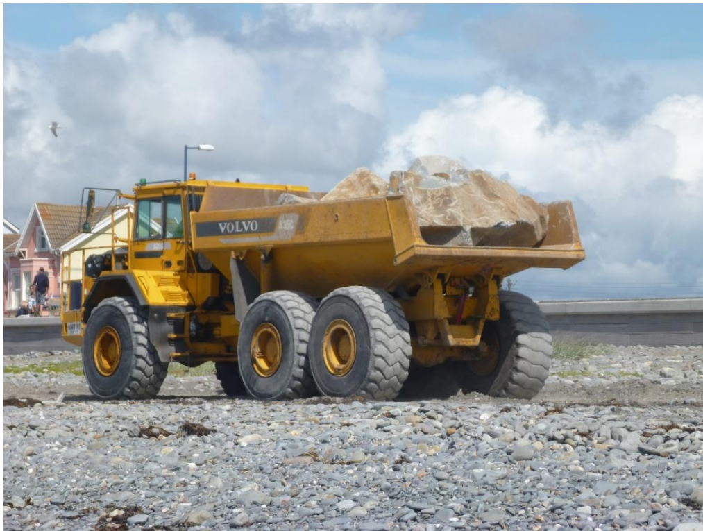
Figure 1-5 - Wheeled Dumper Transporting Rock
