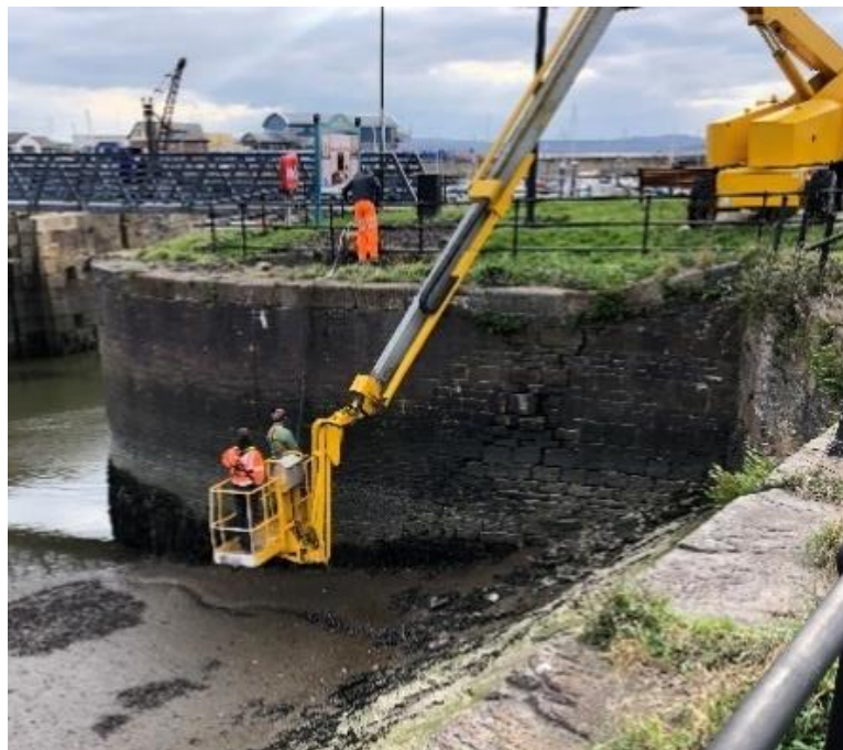
Figure 1-9 - Negative Mobile Elevated Working Platforms (MEWP's) to Repair Walls from Above High Water
