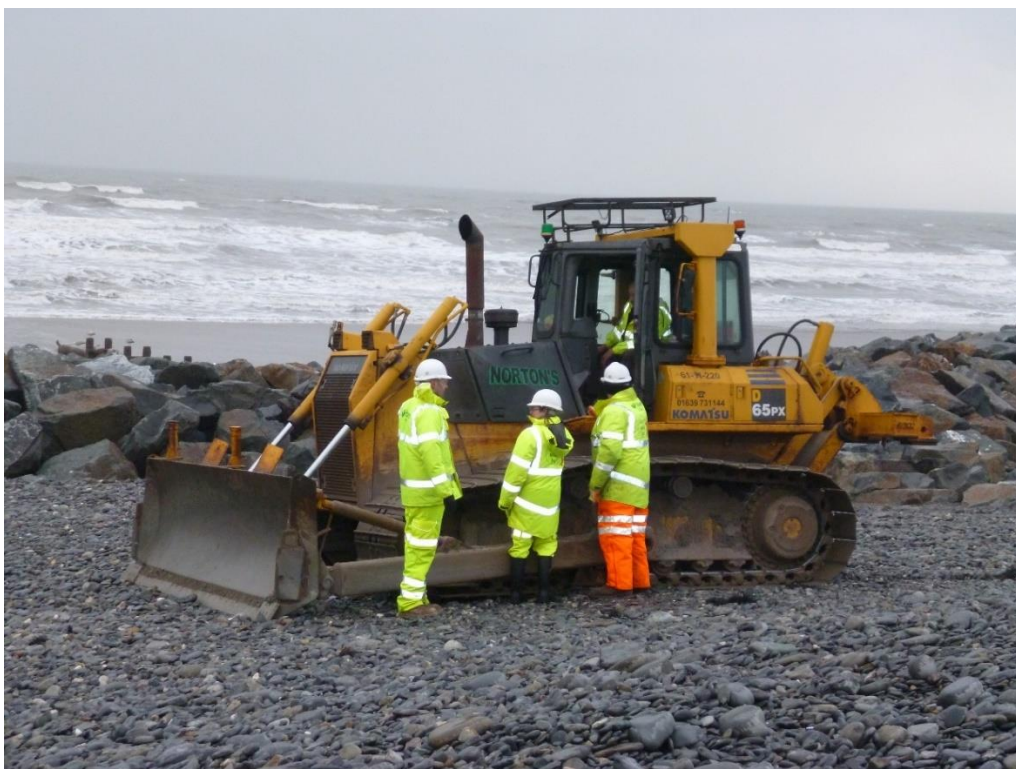
Figure 1-6 - Dozer to Spread out the Imported Shingle
