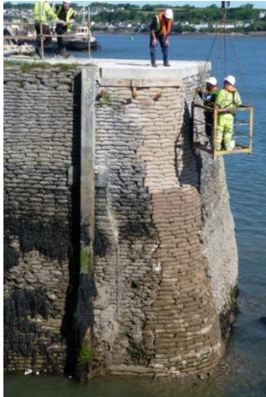
Figure 1-11 - Repointing and Wall Repairs by Rope Access
