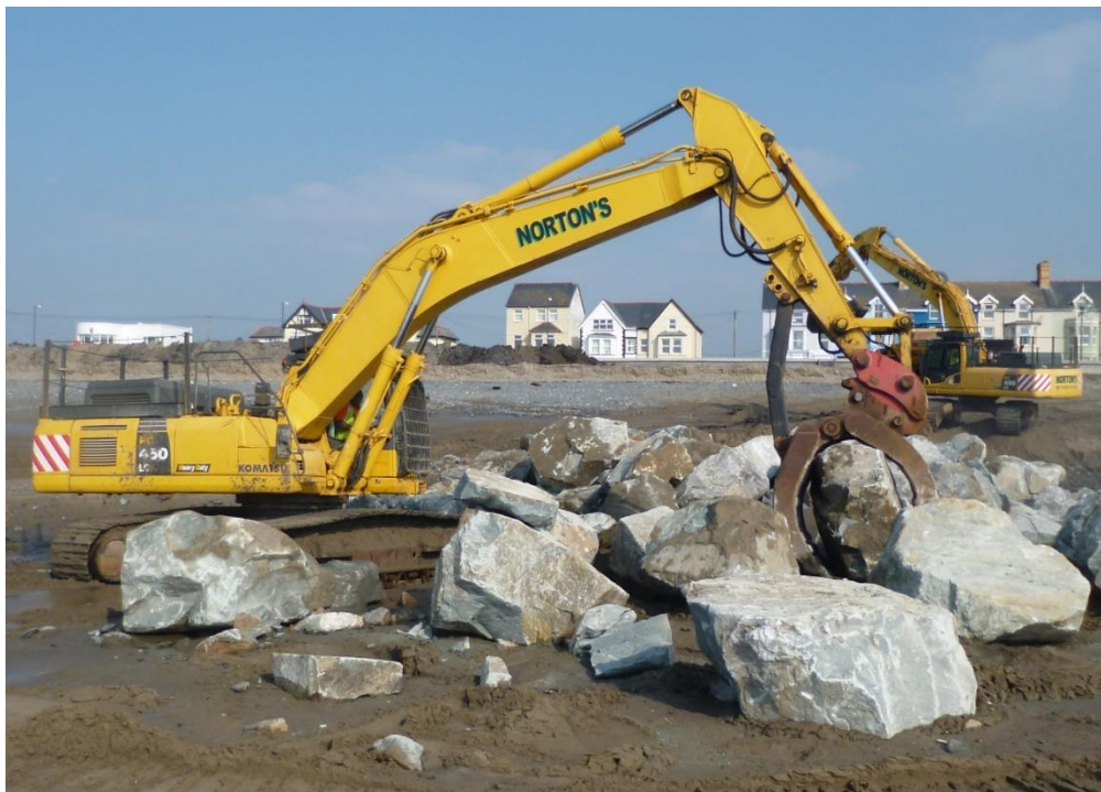
Figure 1-4 - Tracked Excavator with Grab to Pick Up and Place Rock
