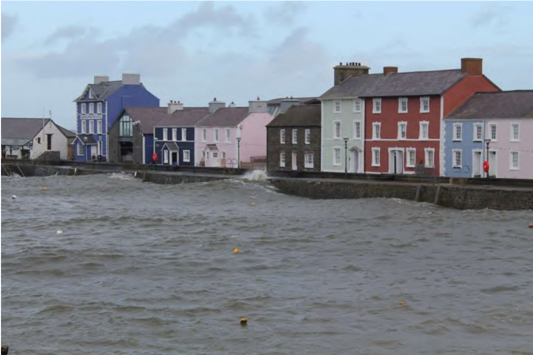
Insert 1-1 Waves overtopping the Northeast Quay (Asset 9) at Quay Parade.
