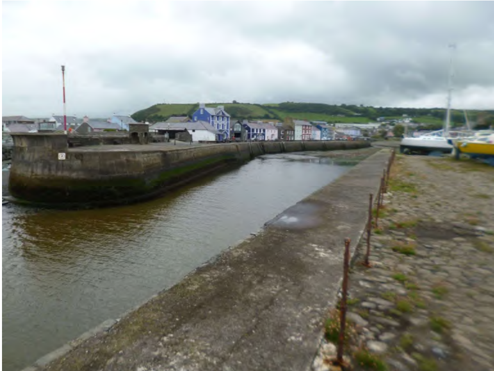
Insert 6-8 View into the Harbour from the South Pier (Asset 9). The North Pier (Asset 7) is visible to the left of this image.
