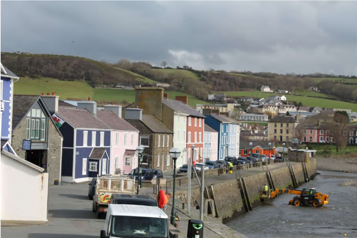
Insert 6-2 Numbers 3-11 Quay Parade (Asset 13) looking southeast
