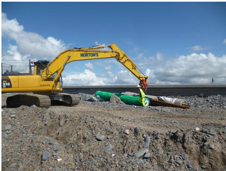
Figure 3-2 - Tracked Excavator Placing Geotextile
