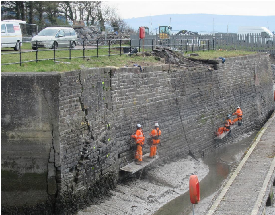
Figure 3-10 - Repointing and Wall Repairs by Rope Access
