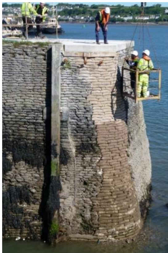
Figure 3-9 - Crane and Basket to Carry Operatives for Wall Repairs
