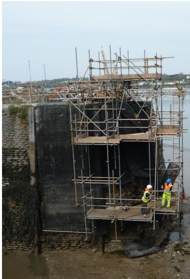
Figure 3-7 - Scaffolding for South Pier and Wall Repairs
