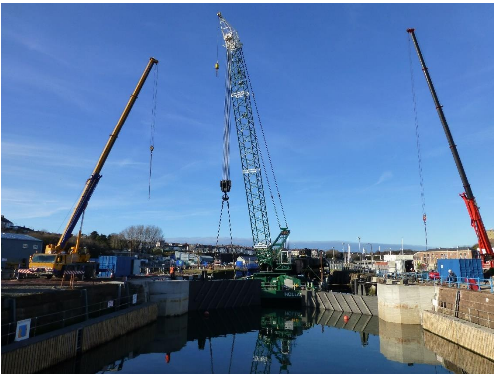
Figure 3-12 Barge, Crane and Gate at Milford Marina
