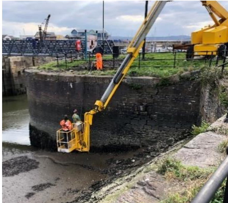
Figure 3-9 - Crane and Basket to Carry Operatives for Wall Repairs
